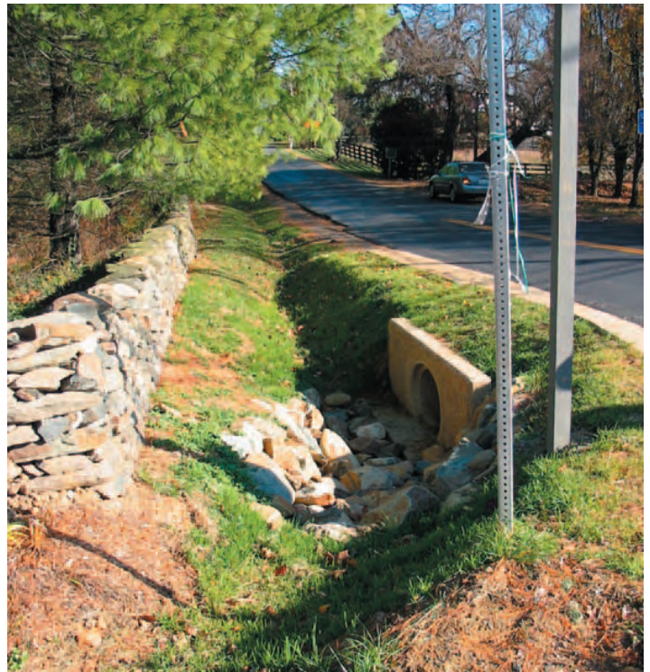
Along Route 50, in Upperville, Virginia, natural field stone was used in lieu of rip-rap and all concrete used for drainage structures incorporated an exposed aggregate finish in order to minimize the contrast with the adjoining stone wall (reconstructed with the same stone as on-site).
