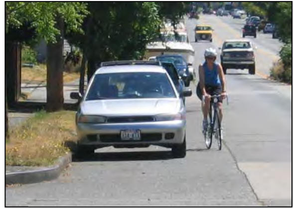
Figure 4.3 Poor Concrete Seam Placement
