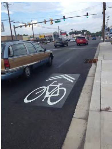
Figure 3.2 Shared Lane Marking (Sharrow) U.S. 113 in Salisbury
