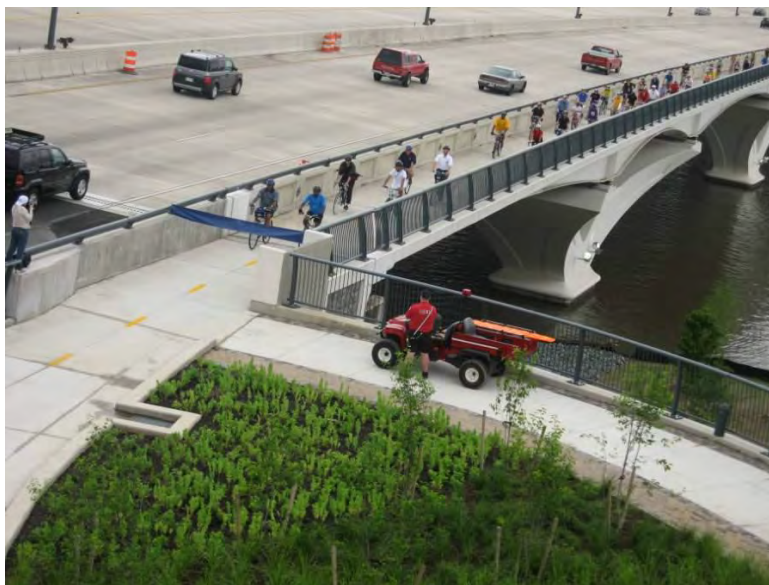
Figure 8.2 Woodrow Wilson Bridge Trail
