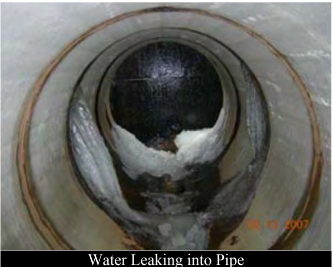
Water Leaking into Pipe
