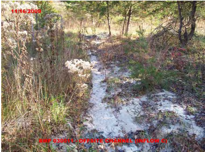
Minor Sediment Accumulation in Inflow Ditch
