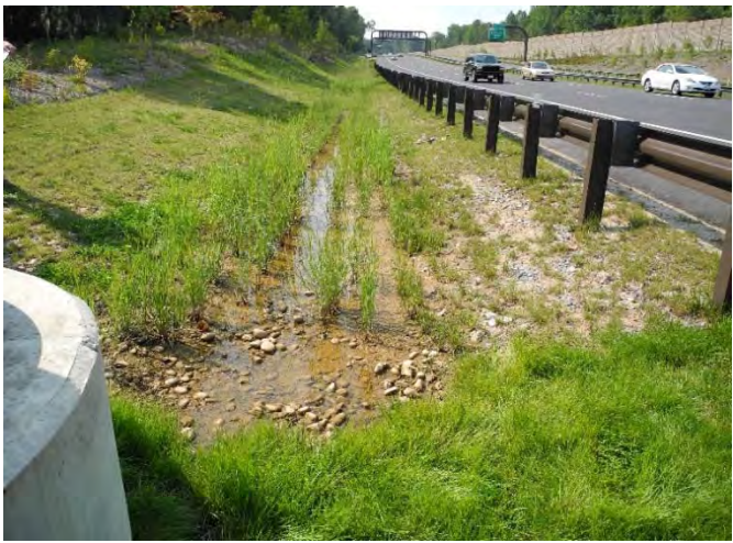
Ponding Water in Bio-Swale
