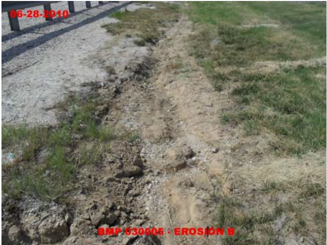
Minor Erosion in Grass Swale
