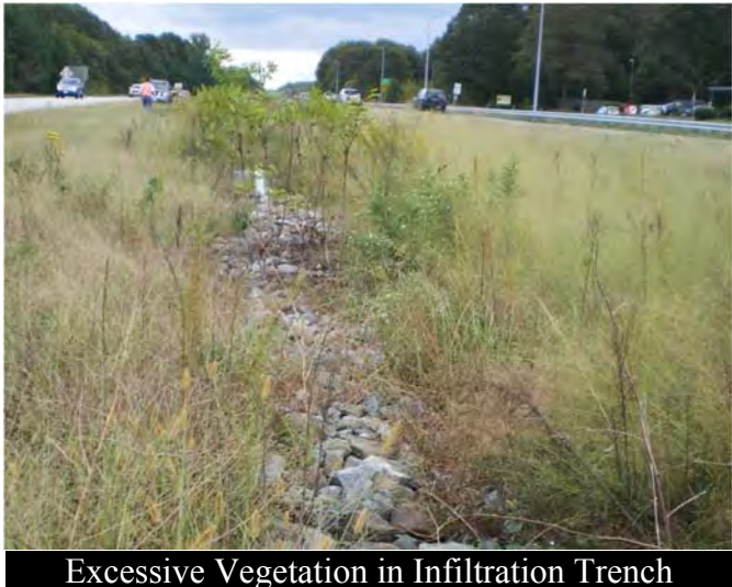
Excessive Vegetation in Infiltration Trench
