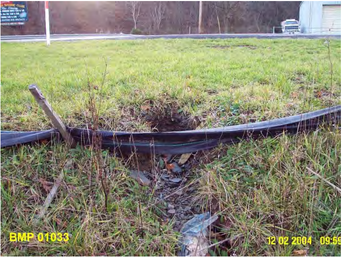
Minor Erosion Under Silt Fence
