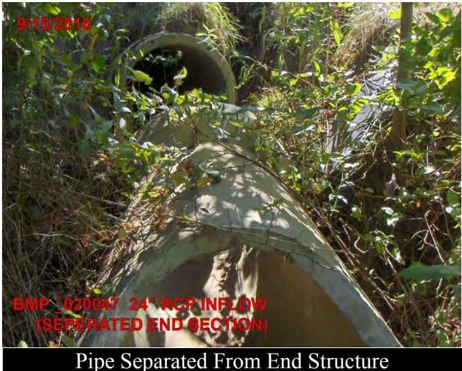
Pipe Separated From End Structure
