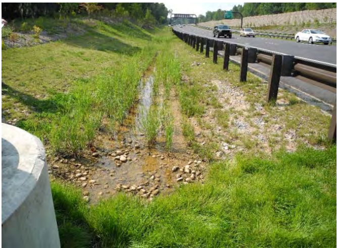
Ponding Water in Bio-Swale
