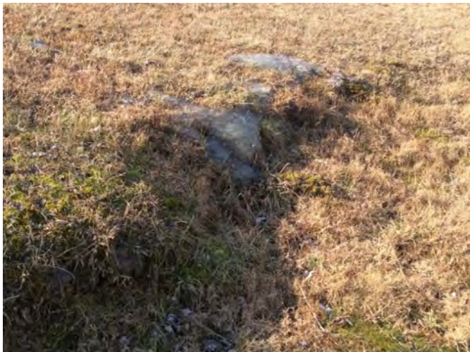
Frozen Seepage Through Embankment
