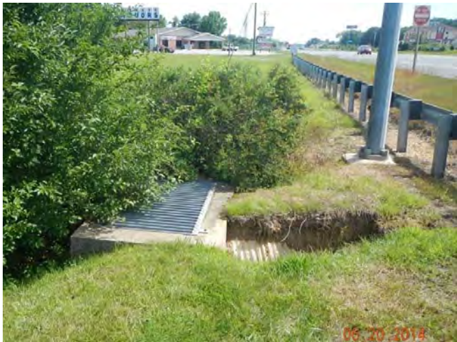
Eroded Embankment Exposing Pipe
