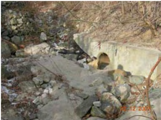
Major Sediment Accumulation at Outfall
