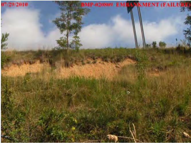
Eroded Embankment
