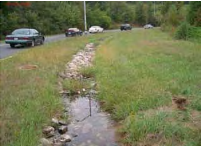
Saturated Infiltration Trench
