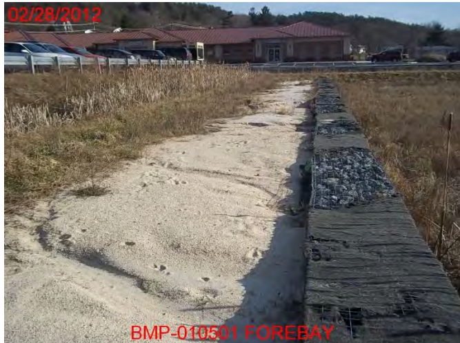
Major Sediment Accumulation in Forebay
