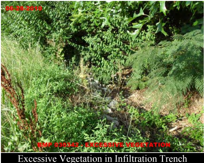
Excessive Vegetation in Infiltration Trench
