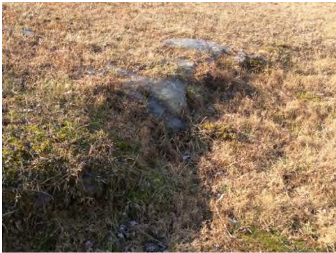
Frozen Seepage Through Embankment
