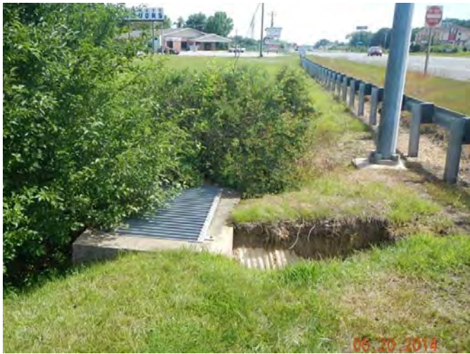
Eroded Embankment Exposing Pipe
