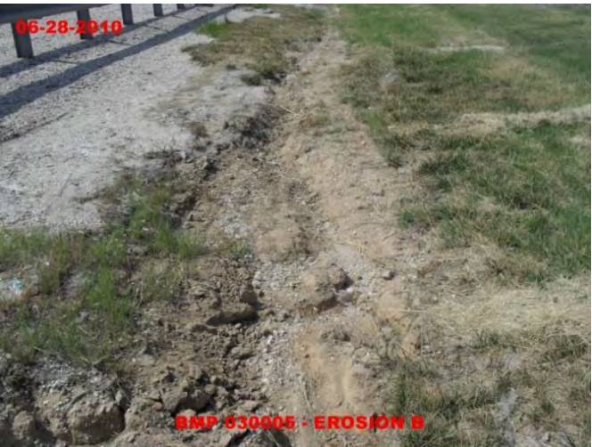
Minor Erosion in Grass Swale
