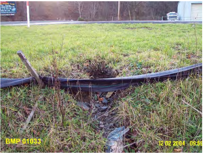
Minor Erosion Under Silt Fence
