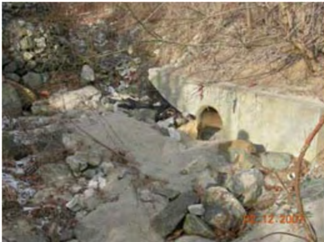
Major Sediment Accumulation at Outfall
