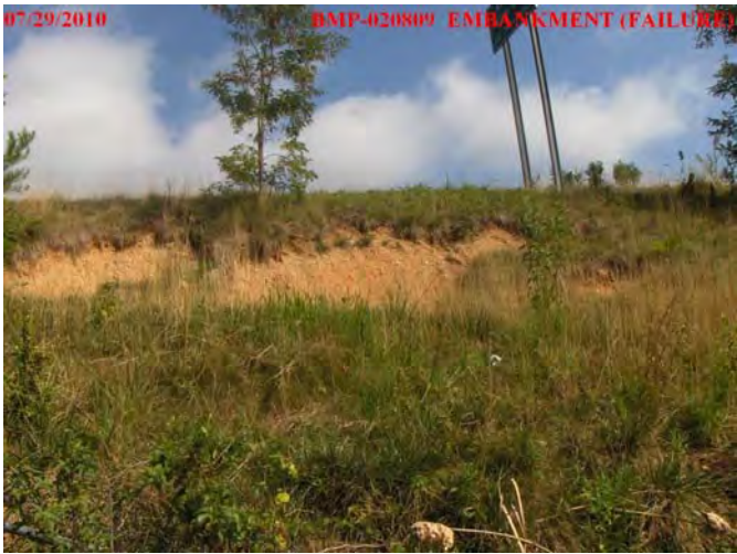
Eroded Embankment
