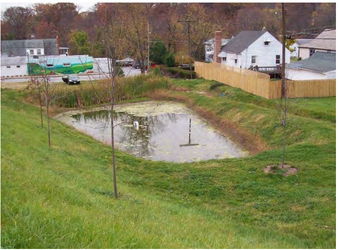
Surface Sand Filter Not Draining
