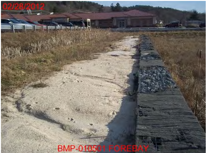
Major Sediment Accumulation in Forebay
