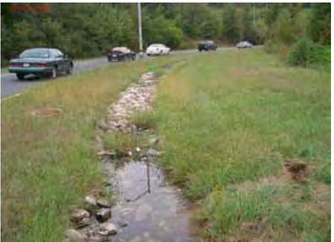
Saturated Infiltration Trench
