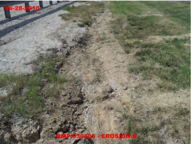
Minor Erosion in Grass Swale
