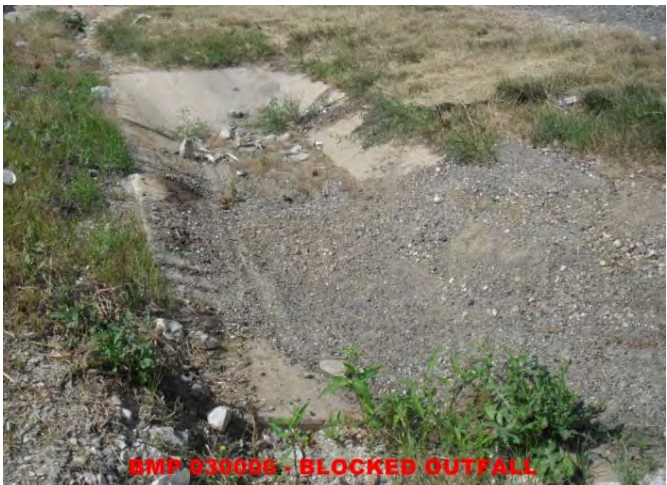
Accumulated Sediment Blocking Outflow Point
