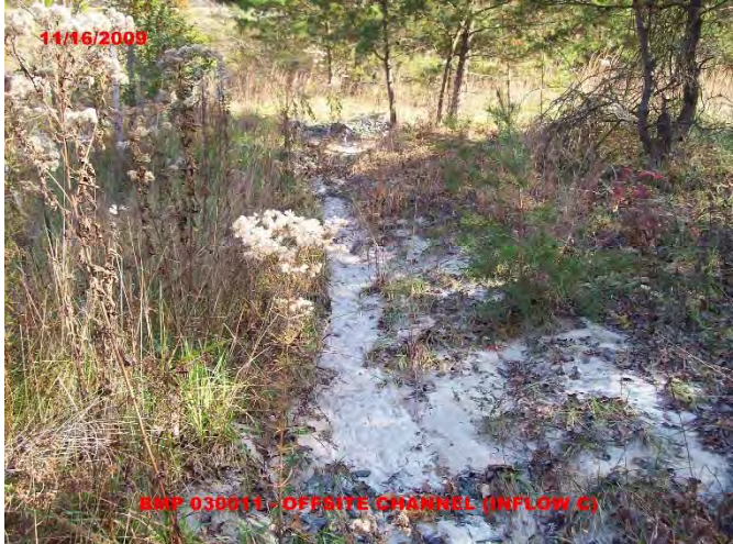
Minor Sediment Accumulation in Inflow Ditch
