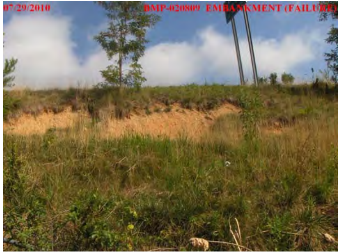
Eroded Embankment
