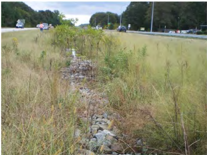
Excessive Vegetation in Infiltration Trench
