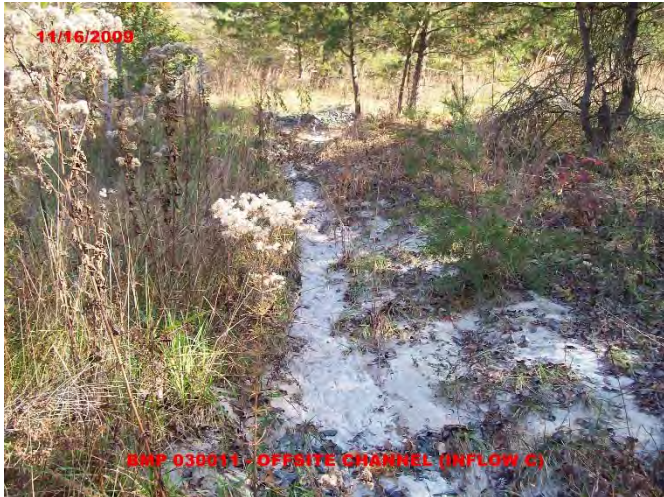
Minor Sediment Accumulation in Inflow Ditch
