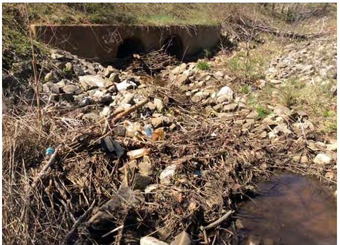
Accumulated Debris Blocking Outflow Point
