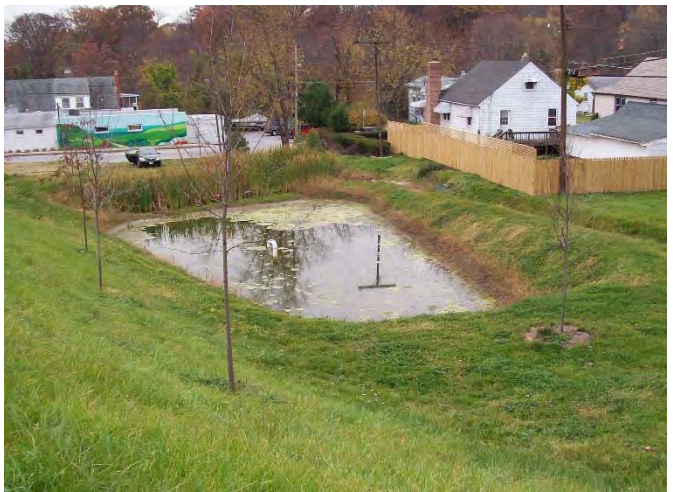
Surface Sand Filter Not Draining
