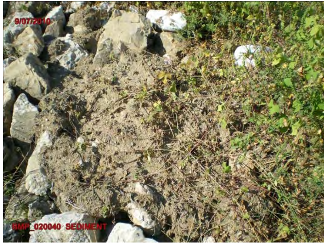
Minor Sediment Accumulation
