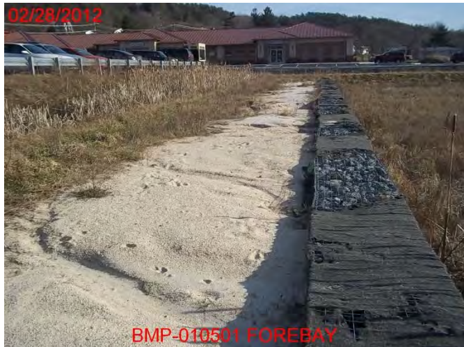
Major Sediment Accumulation in Forebay
