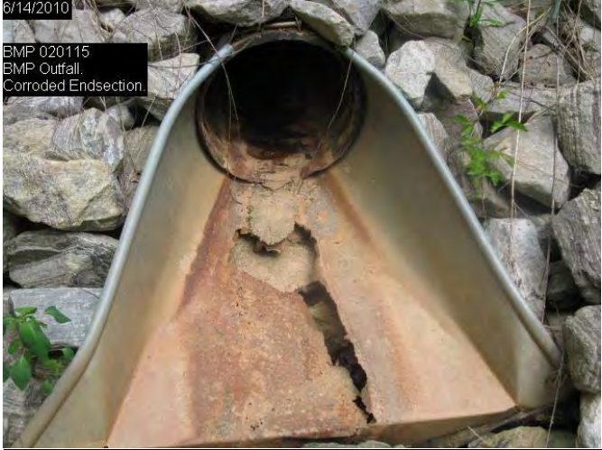
Deteriorated CMP End Structure
