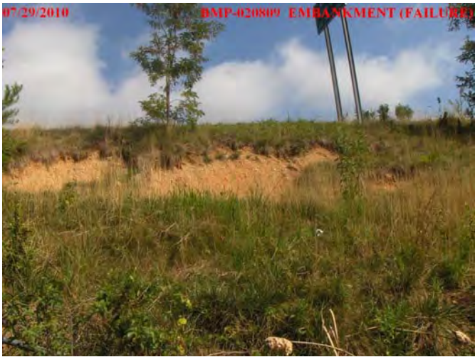
Eroded Embankment
