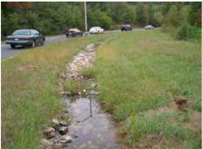
Saturated Infiltration Trench
