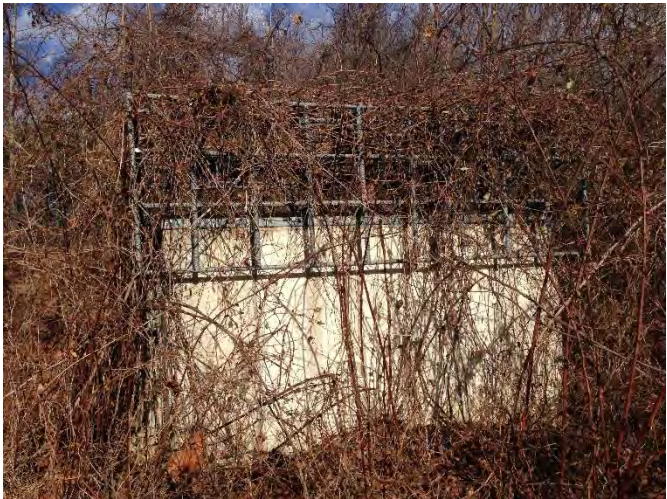
Vegetation Obstructing Riser Structure
