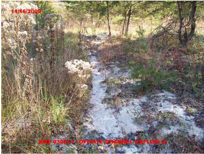
Minor Sediment Accumulation in Inflow Ditch
