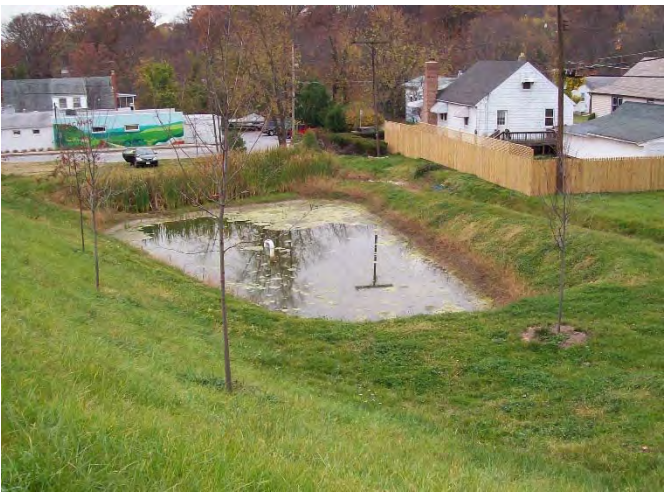
Surface Sand Filter Not Draining
