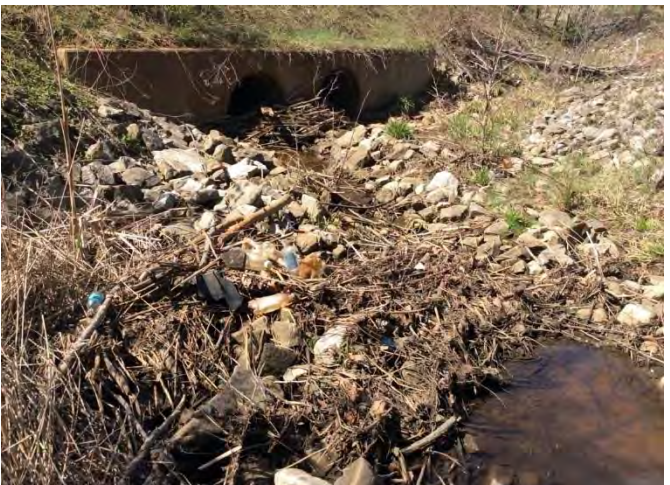
Accumulated Debris Blocking Outflow Point
