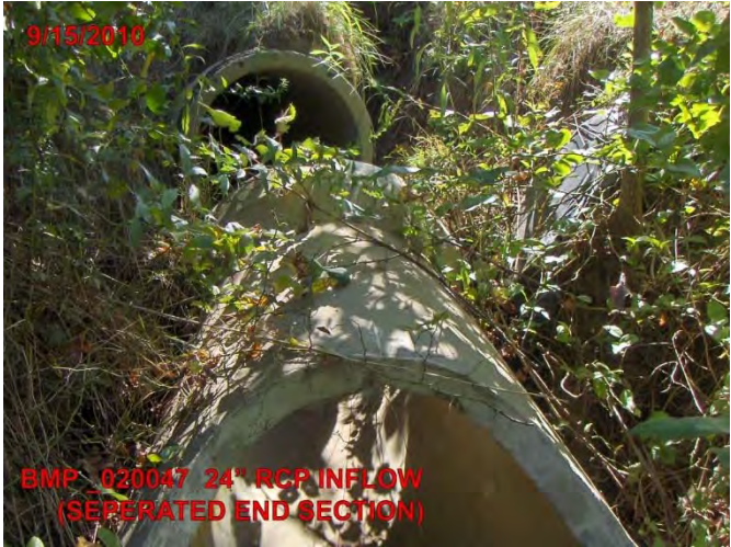
End Structure Separated From Pipe
