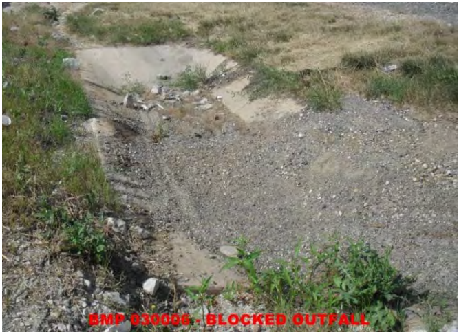
Accumulated Sediment Blocking Outflow Point
