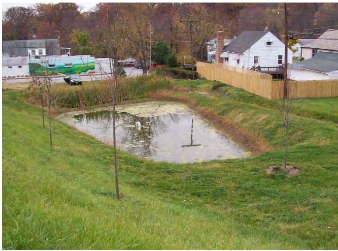
Surface Sand Filter Not Draining
