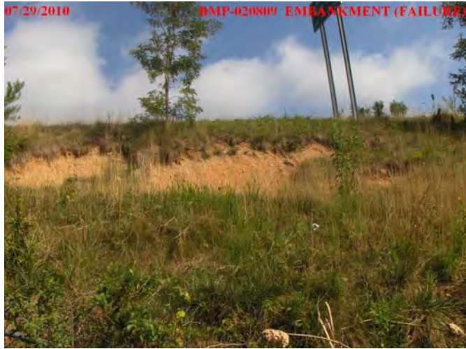
Eroded Embankment
