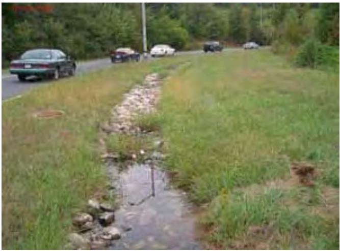
Saturated Infiltration Trench
