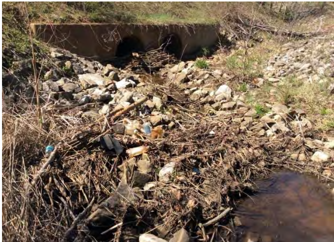
Accumulated Debris Blocking Outflow Point
