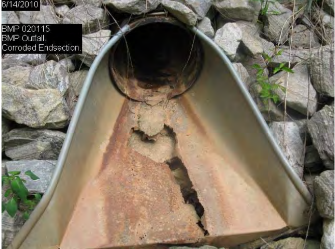
Deteriorated CMP End Structure
