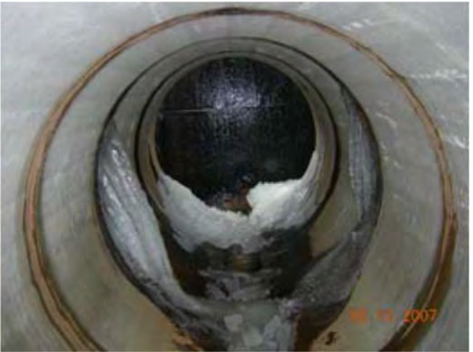
Water Leaking into Pipe
