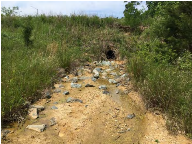
Major Sediment Accumulation at Outfall
