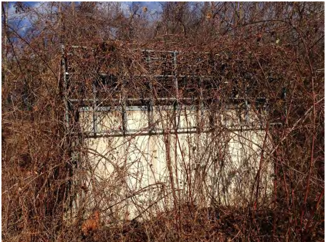
Vegetation Obstructing Riser Structure
