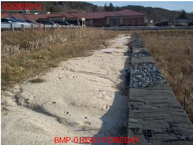
Major Sediment Accumulation in Forebay
