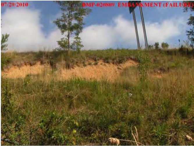
Eroded Embankment
