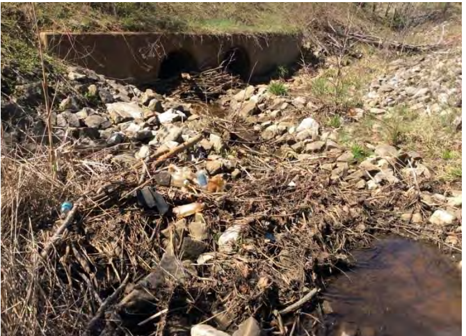
Accumulated Debris Blocking Outflow Point
