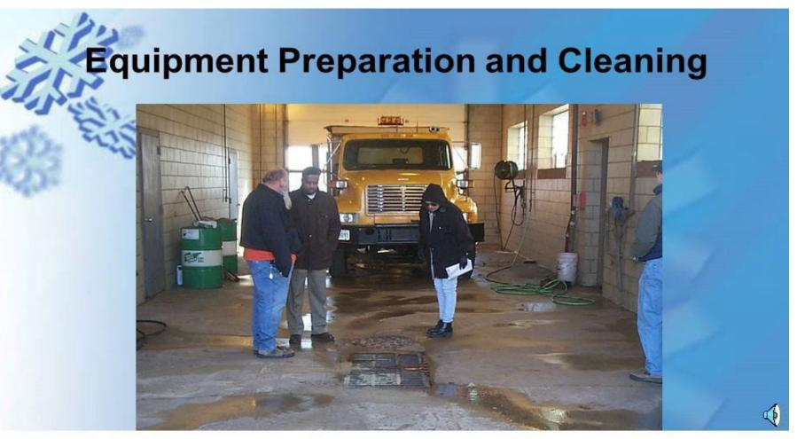
Clean equipment in wash bay so that wash water is treated by the grit separator and oil/water separator to minimize the discharge of sediment, salt and heavy metals into the environment.
