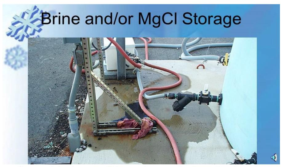
Inspect tanks monthly paying particular attention to valves and fittings. Place drip pan under leaks and repair immediately.
