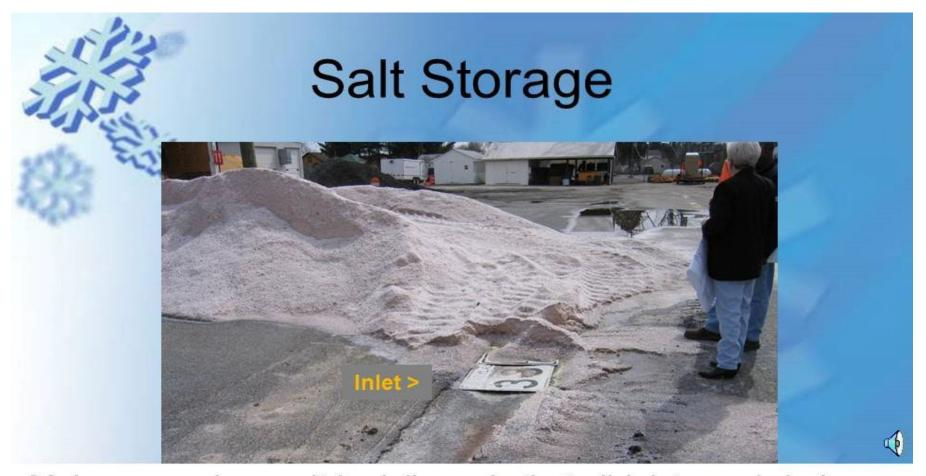
Make sure when salt is delivered, that all inlets and drainage structures are protected and all the salt is under covered storage by day's end. Here an inlet was protected by covering it with sheet signing, but overnight rain washed dissolved salt into the drainage system discharging it off site.
