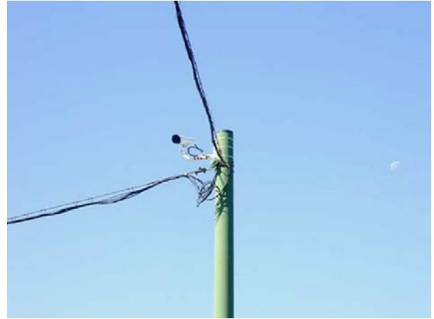
Figure 56 – Typical Video Detection Location (Extension Arm Mount)
