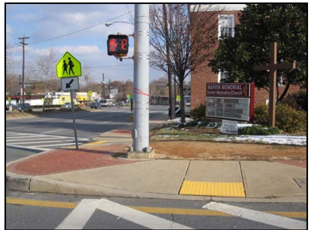
Figure 48 – Countdown Pedestrian Signal and Detectable Warning Surface
