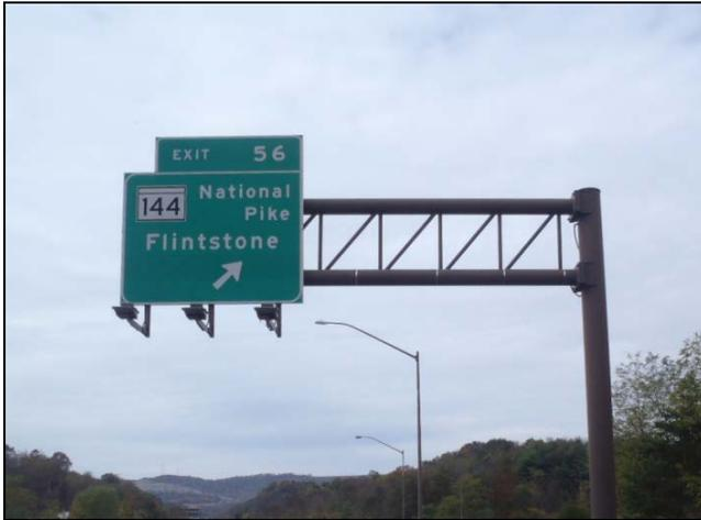
**Figure SN.12 - Sign Lighting Individual Supports**
