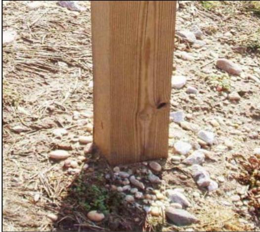
Figure SN.24 - Non-Breakaway Wood Support
