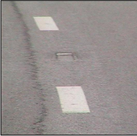
**Figure SN.46 - Recessed Pavement Marker (RPM)**
