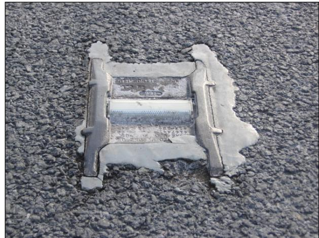
**Figure SN.45 – Snowplowable Raised Pavement Marker**
