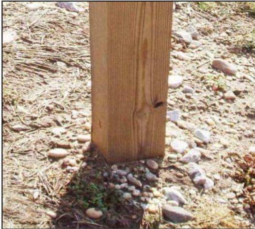
Figure SN.24 - Non-Breakaway Wood Support
