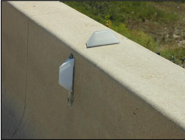
**Figure SN.41 - Top and Side Mounted White Barrier Wall Markers**
