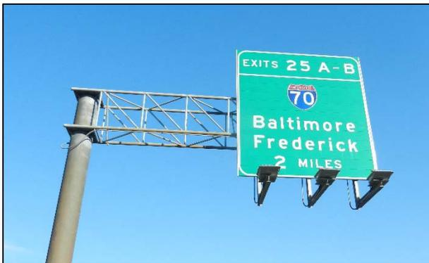
**Figure SN.16 - Typical Box Truss Cantilever**
