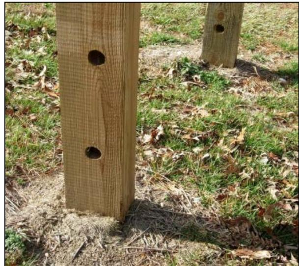
**Figure SN.23 - Breakaway Wood Support**
