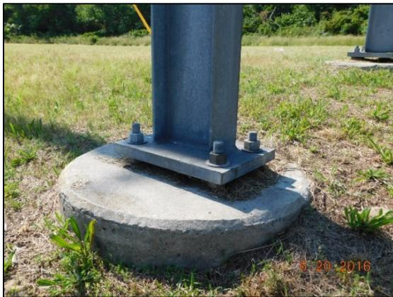
Figure SN. 25 - Non-Breakaway Steel Support
