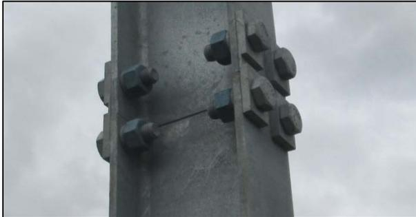
**Figure SN.32 - Breakaway Hinge for Steel Support**
