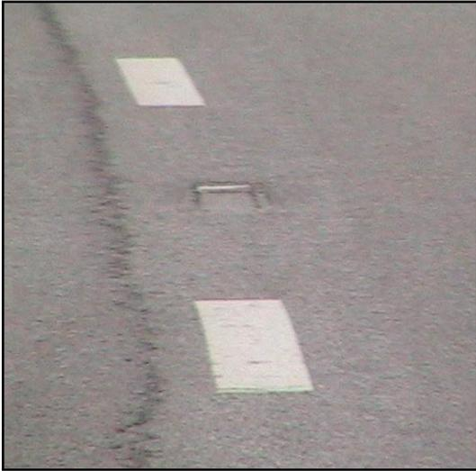
**Figure SN.46 - Recessed Pavement Marker (RPM)**
