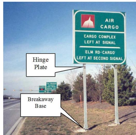
Figure SN.31 - Breakaway Steel Support
