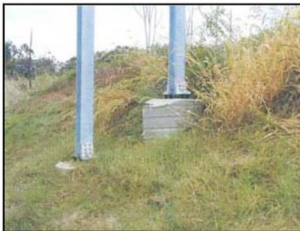
**Figure SN.33 - Improper Supports on Steep Slopes**
