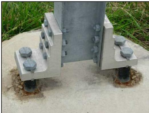
Figure SN. 26 - Breakaway Steel Support
