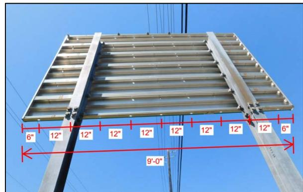
Figure SN.2 - Extruded Aluminum Sign Width
