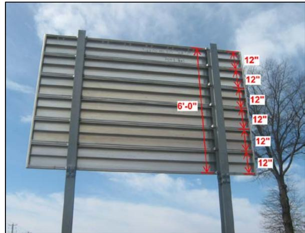
Figure SN.1 - Extruded Aluminum Sign Height
