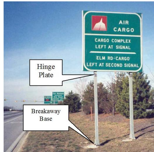
Figure SN.31 - Breakaway Steel Support
