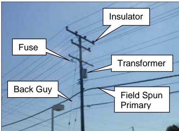
**Figure SG. 3 - Typical Utility Pole Components**
