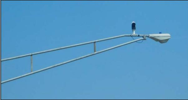
**Figure SG. 24 - Typical Video Detection Location (Lighting Arm Mount)**
