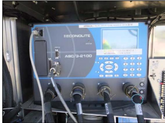
**Figure SG. 36 - Signal Controller**
