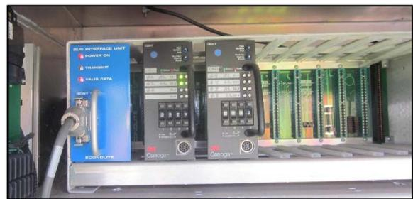
**Figure SG. 40 - 4-Channel Vehicle Detector Amplifiers**
