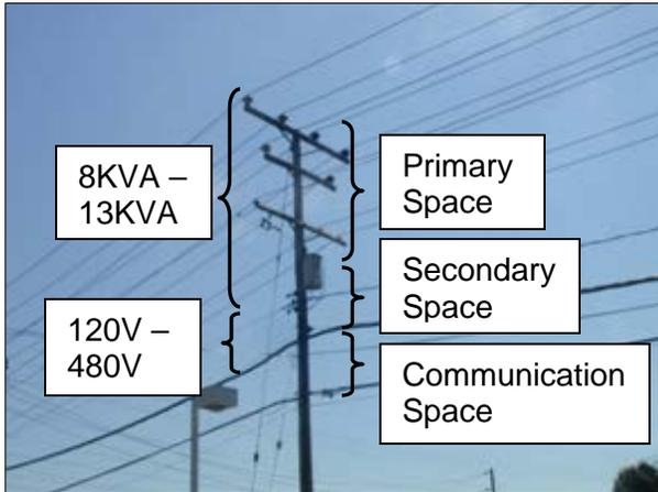
**Figure SG. 2 - Typical Utility Pole "Spaces"**
