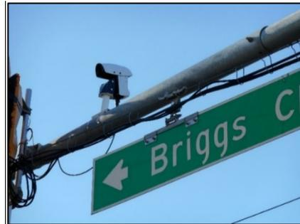
**Figure SG. 23 - Typical Video Detection Location (Mast Arm Mount)**
