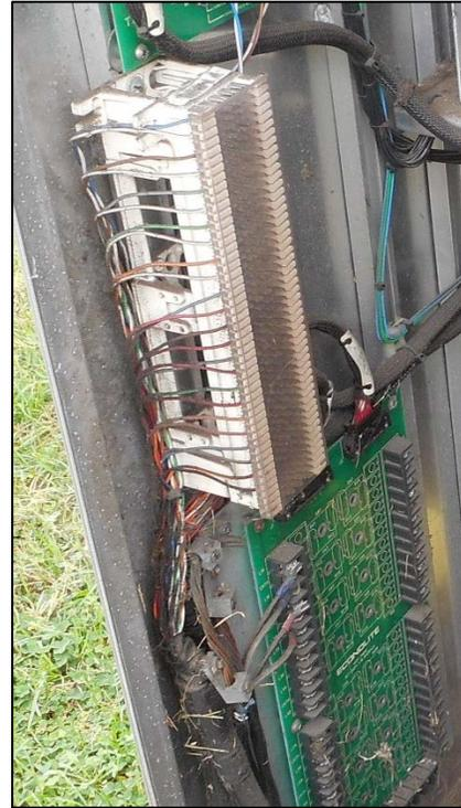
**Figure SG. 41 - 12-Pair Interconnect Cables**
