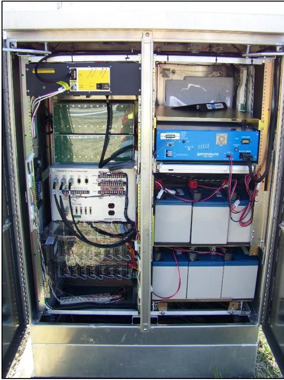
**Figure SG. 39 - Typical Signal Cabinet with UPS (Size 'S')**
