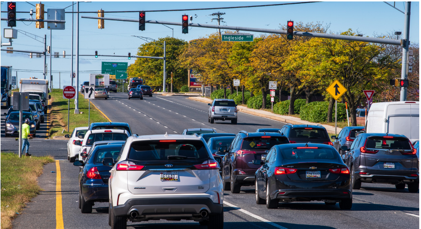
US 40 at Ingleside Avenue Adaptive Signal System
