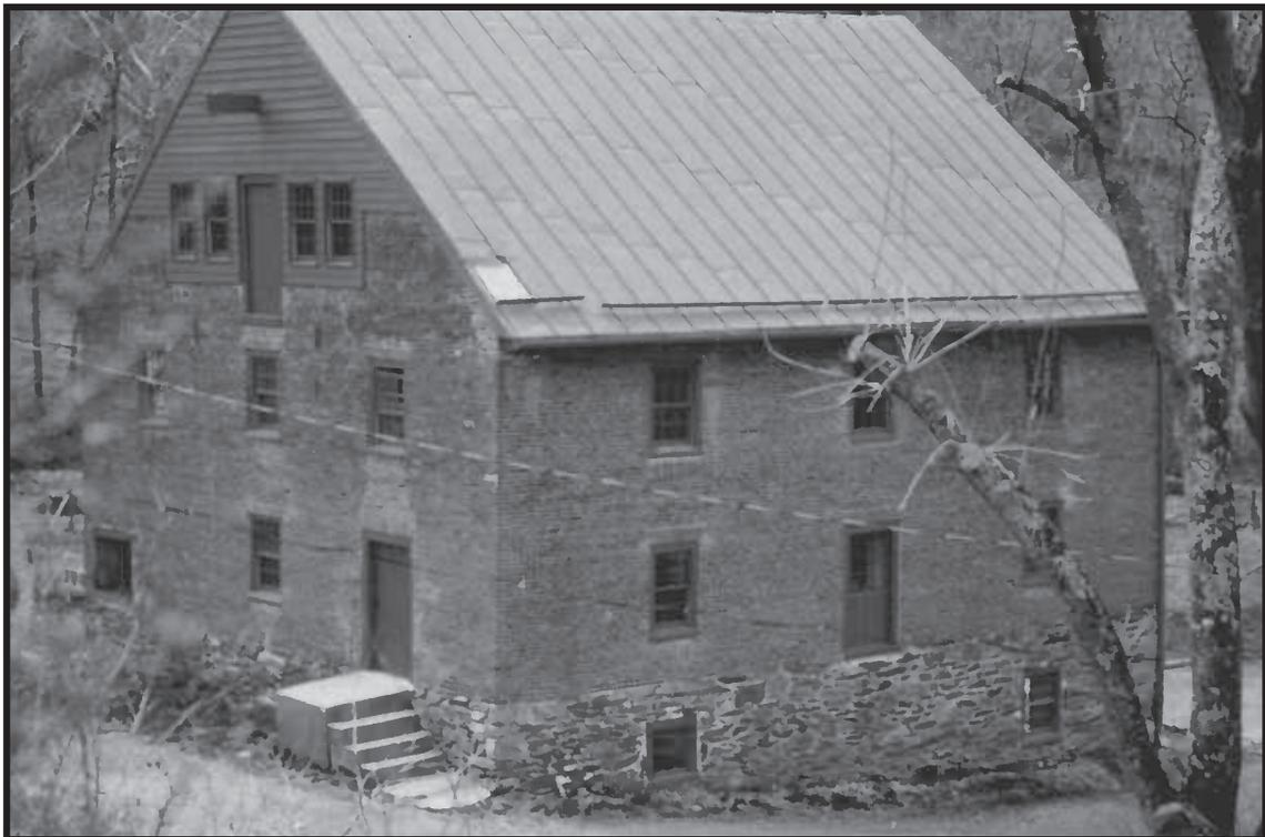
Figure 8: Lewis Mill, Frederick County, Maryland. Similar to the Rice Mill, the Lewis Mill is a two-story brick building with a coursed rubble stone foundation (Source: National Register of Historic Places, Lewis Mill Complex).
