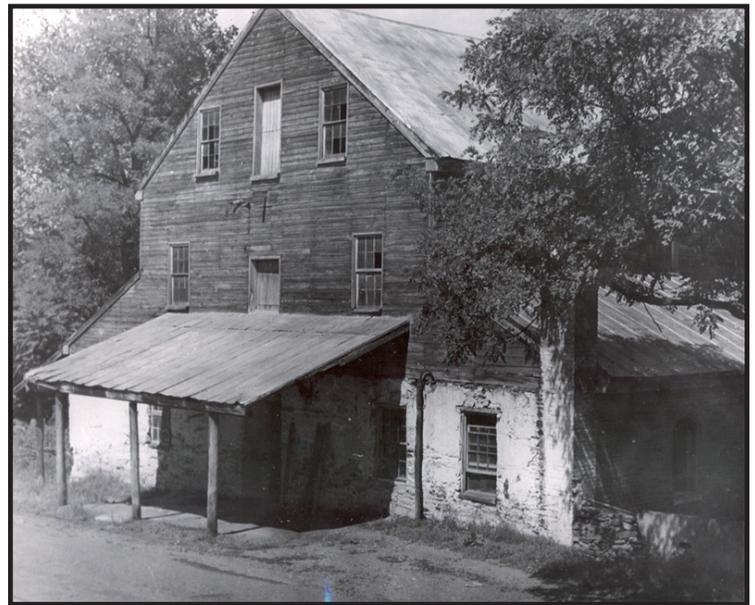
Figure 6: Michael's Mill, Frederick County, Maryland. The mill shows typical eighteenth-century architecture with its gable roof, three bay width, and doors on each story. The weatherboard siding, however, was atypical for Frederick County. (Courtesy of the Frederick County Public Library).
