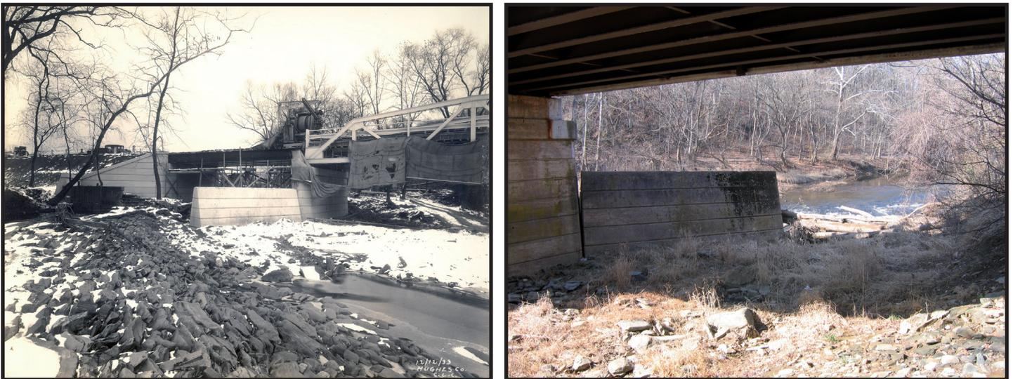
Figure 31 and 32: 1933 Photograph of construction of Bridge No. 1009100 by Hughes C.L.C. Photographers for State Road Commissioners, showing race gate walls and mill dam (left) and race gate on Pier D, view west, 2008 (Courtesy of the State Highway Administration).
