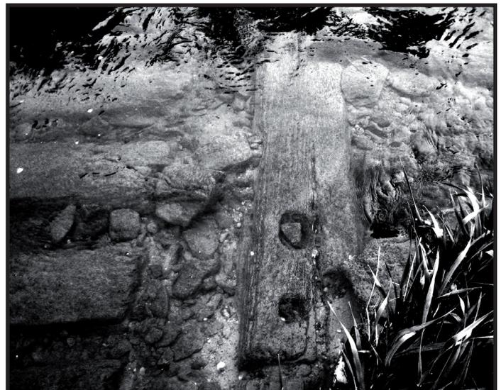
Figure 30: Remaining underwater frame cribbing from the no longer extant dam, 2008 (Courtesy of State Highway Administration).
