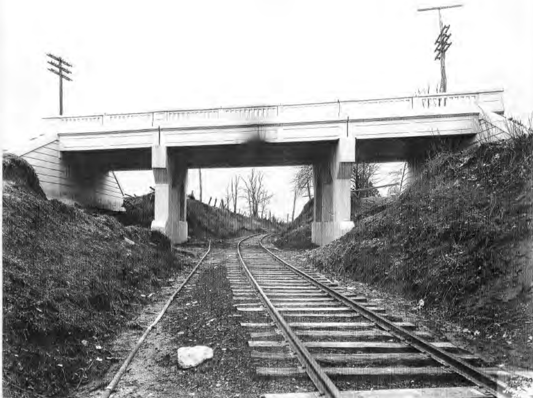
PLATE 15: Typical Concrete Multiple-Span Beam Bridge: Bridge Crossing Railroad Tracks at Fallston
