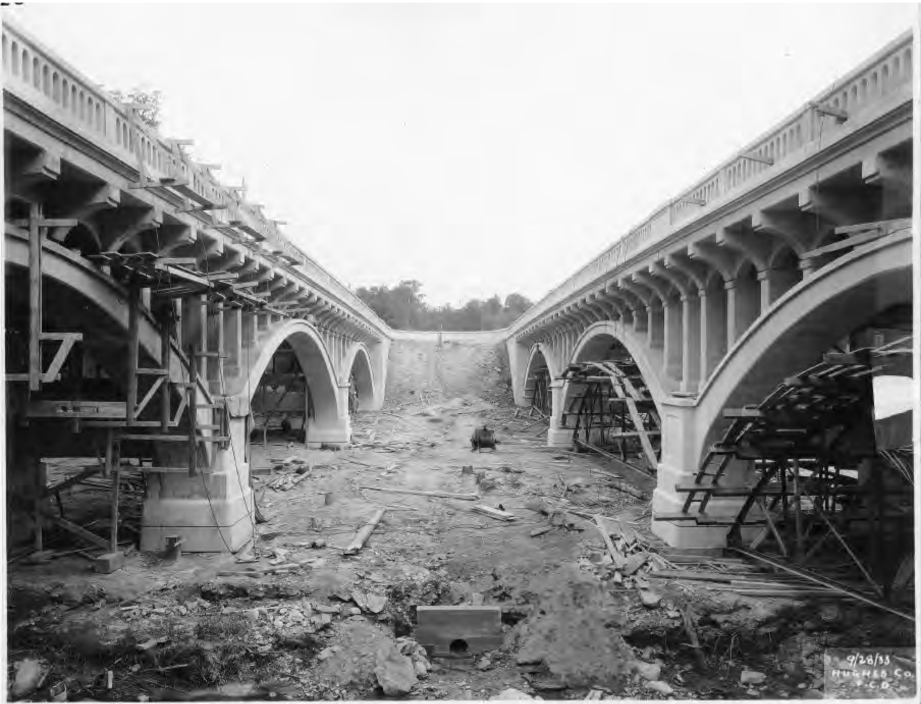
PLATE 14: Typical Concrete Open Spandrel Bridges Under Construction: Bridges on Loch Raven Boulevard in Baltimore
