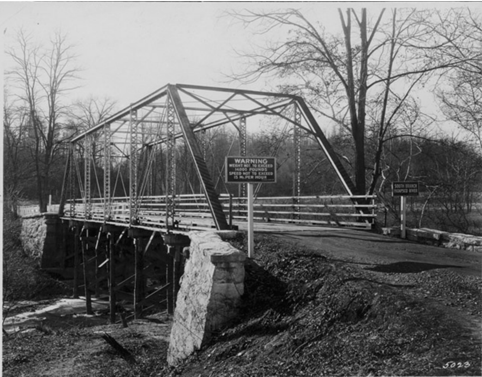
PLATE 5: Typical Metal Pratt Through Truss Bridge: Bridge Crossing the South Branch of the Patapsco River at Henryton
