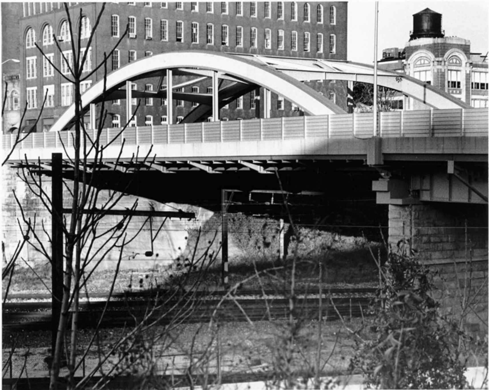
PLATE 12: Typical Metal Arch Bridge: Bridge on Guilford Avenue in Baltimore
