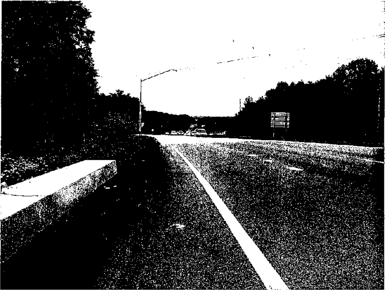
5) View east. Shows MD 198 bridge.
