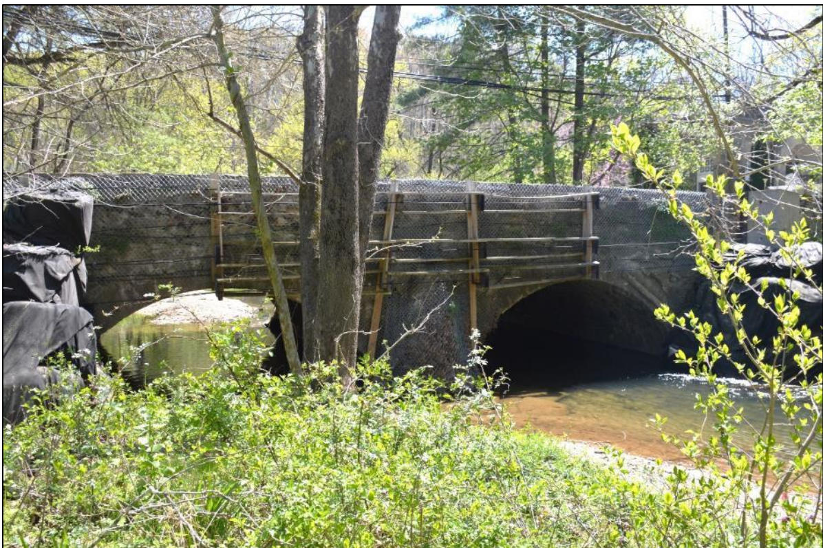
Photo 3: Emergency chain-link netting and timber bracing on west/upstream spandrel walls and pier, view south. Note fabric covered blocks at upstream abutments.
