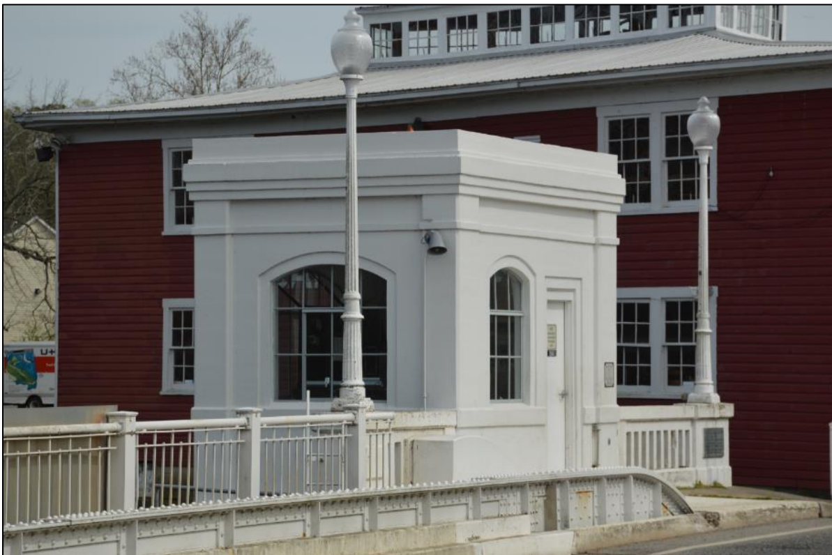
Photo 3: Detail of Tender's House, with original lighting, concrete parapet, metal railing, and bascule girder, view east.
