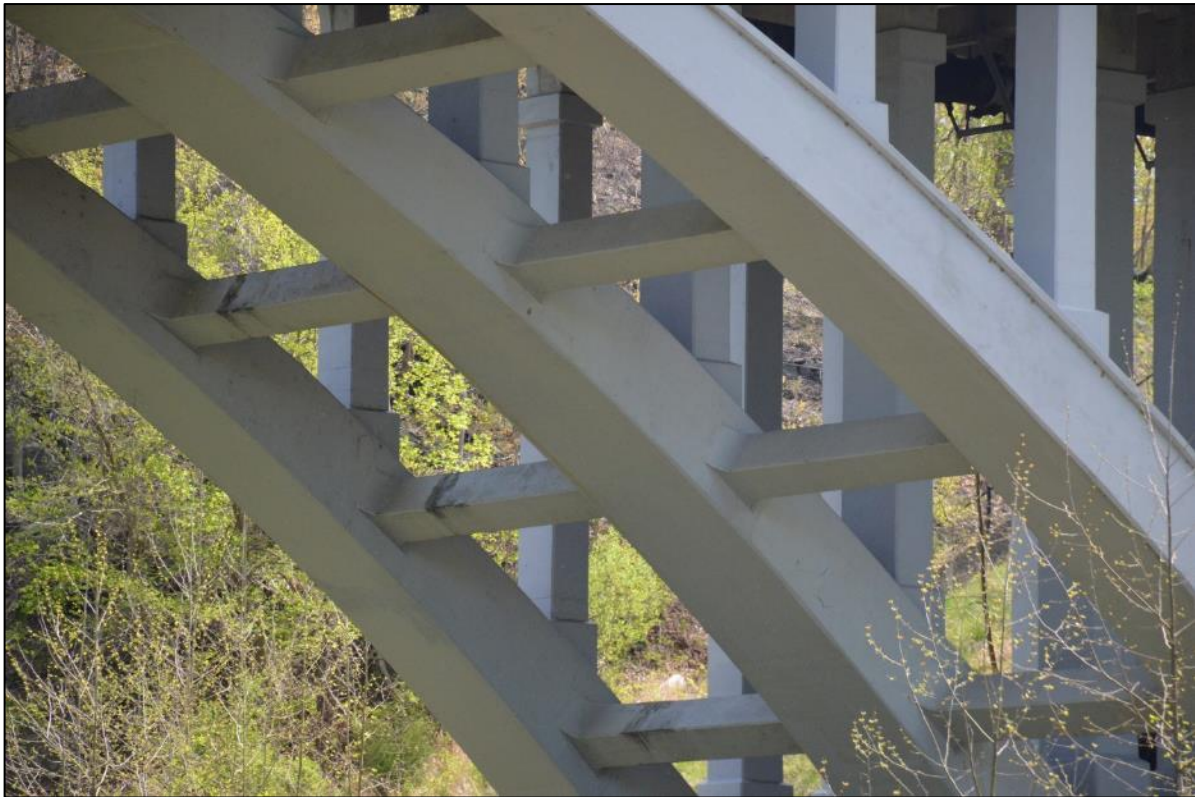
Photo 3: Detail repaired arch ring and new struts.
