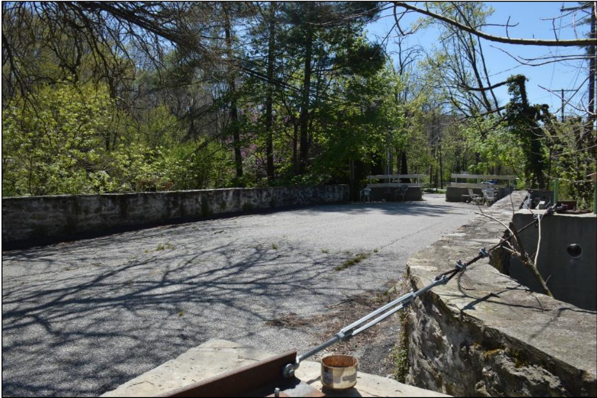
Photo 2: View of bridge deck showing emergency repair measures in foreground, view south. Bridge is closed to traffic.
