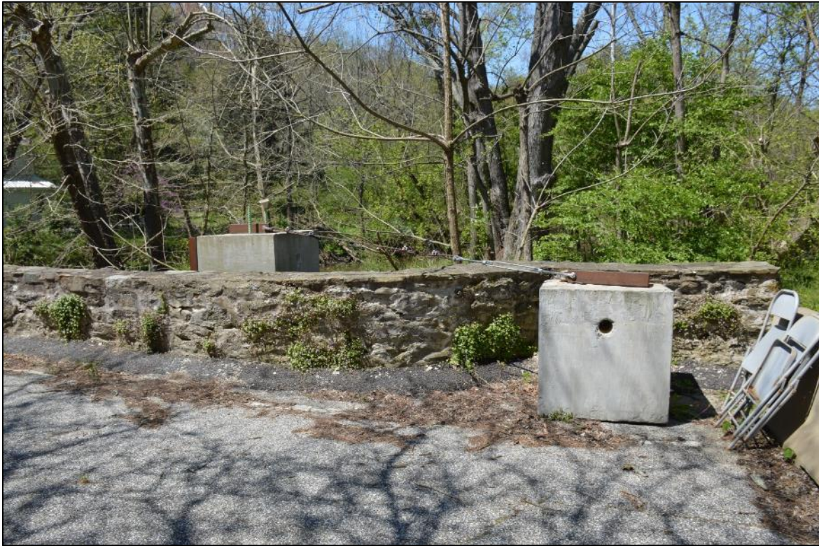
Photo 4: Detail of tension rod/cable system with deadmen anchor at northeast approach. Similar anchorage is present at southwest end of bridge deck. View northwest.
