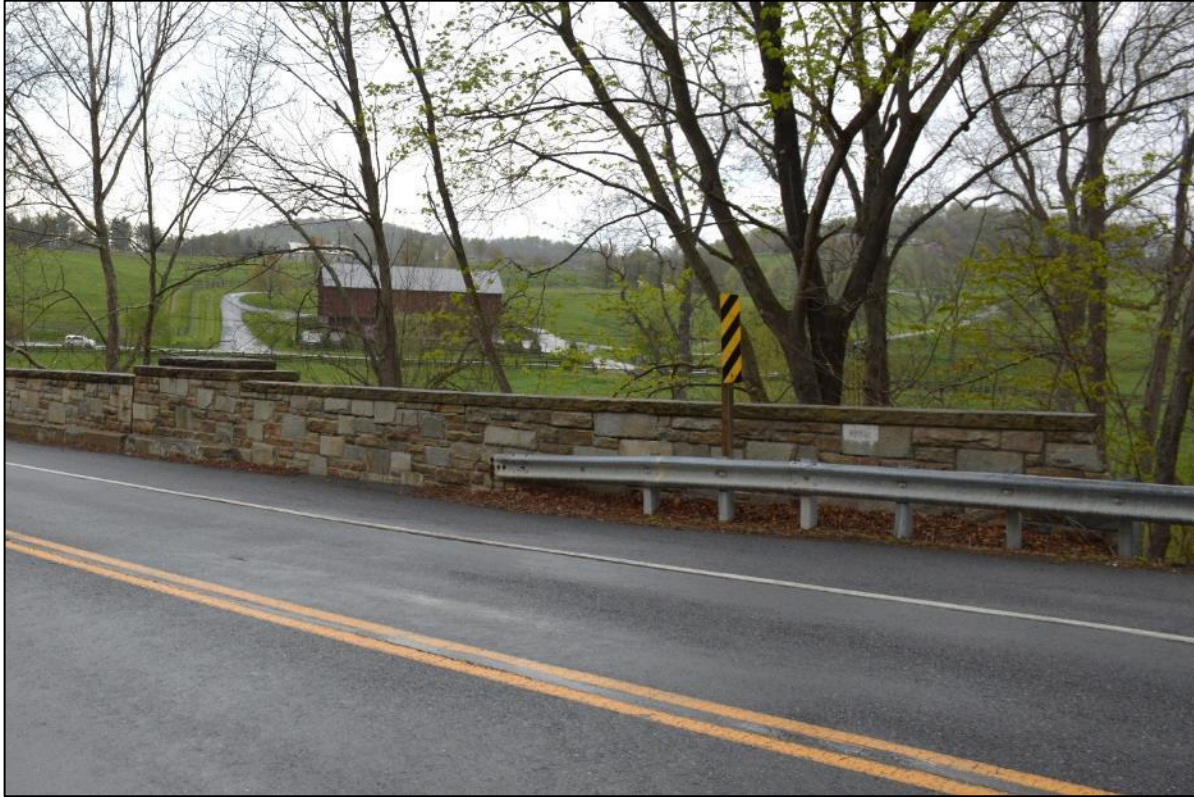
Photo 2: Northeast parapet with attached w-beam guardrail. Note proximity of trees, view north.
