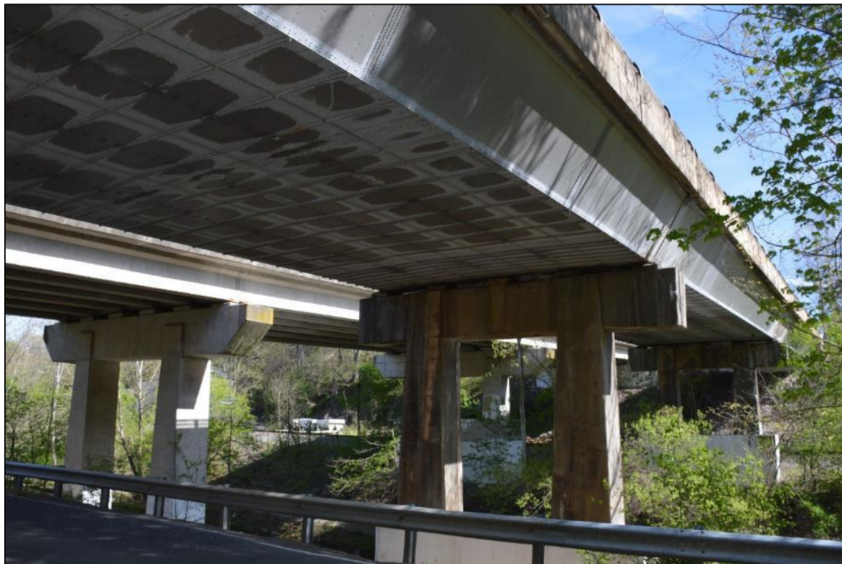
Photo 1: Bridge from River Road, Span 3 in foreground, view north. Note box girder profile and vegetation. Patapsco River (Span 2) and CSX Railroad (Span 1) in distance.
