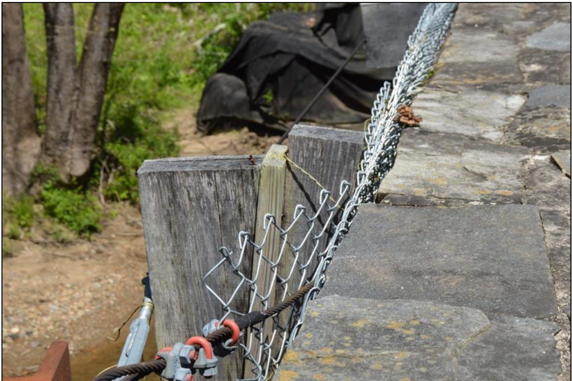
Photo 5: Detail of emergency repair. Note chain-link netting suspended from cable and held in place against spandrel wall by timber bracing secured and tightened by threaded rod and turnbuckles.
