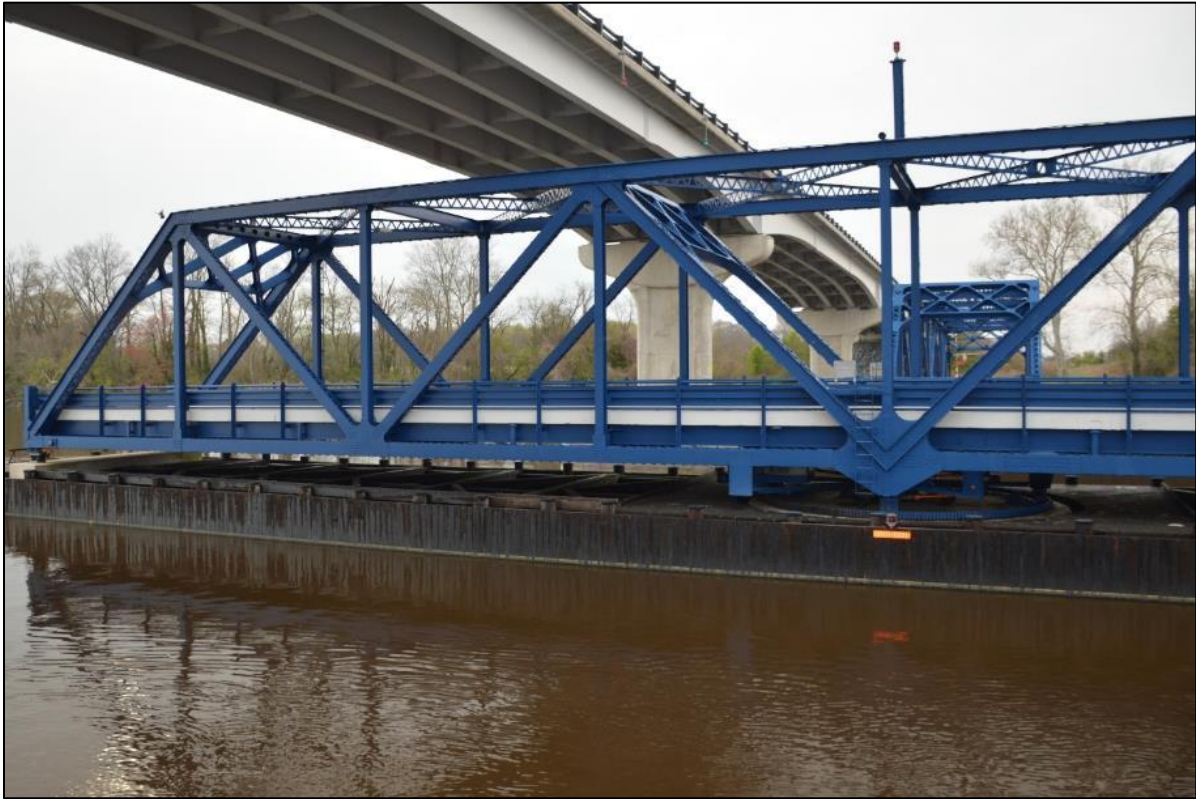
Photo 2: Swing span resting in open position with new bridge overhead, view north.
