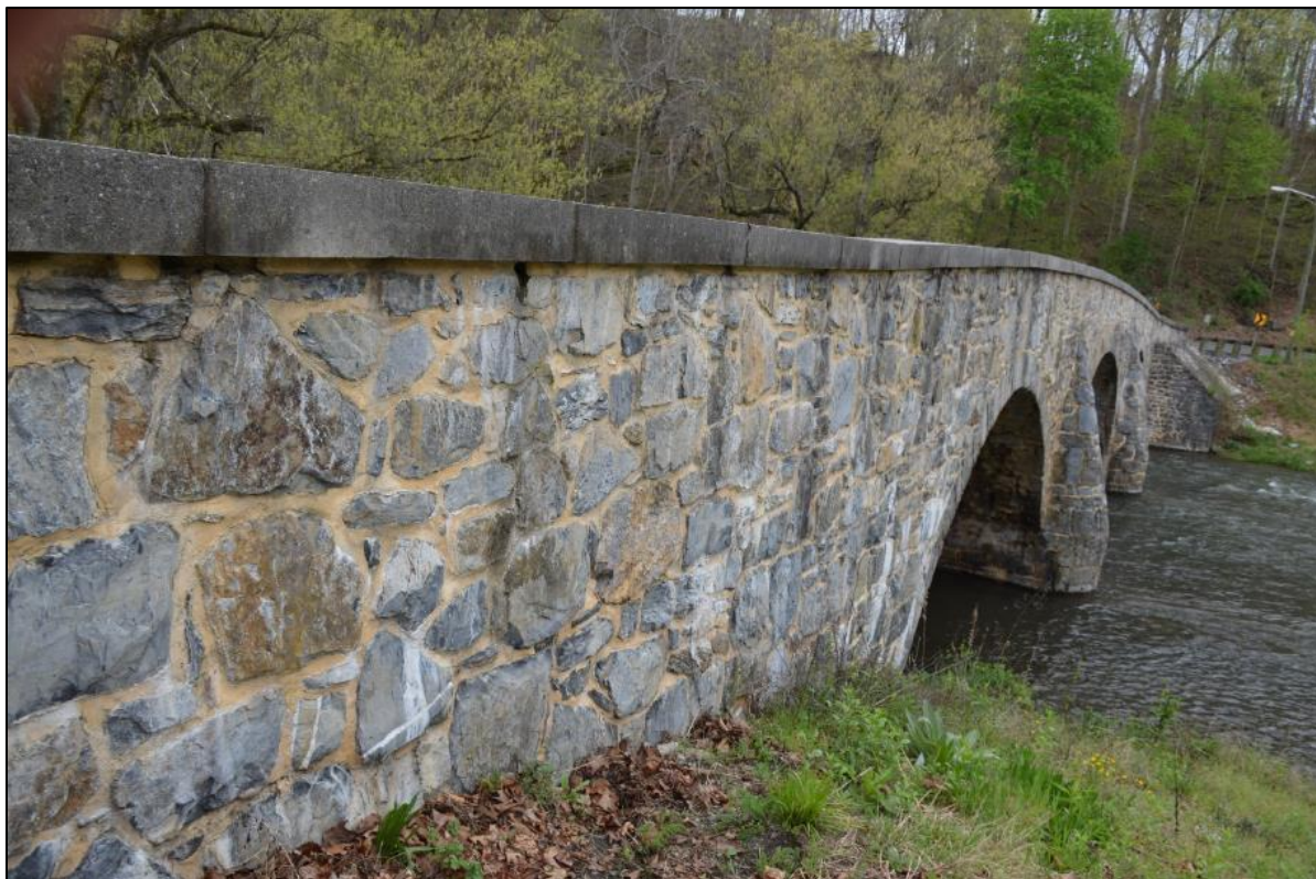
Photo 3: Detail of downstream parapet with concrete parapet caps.
