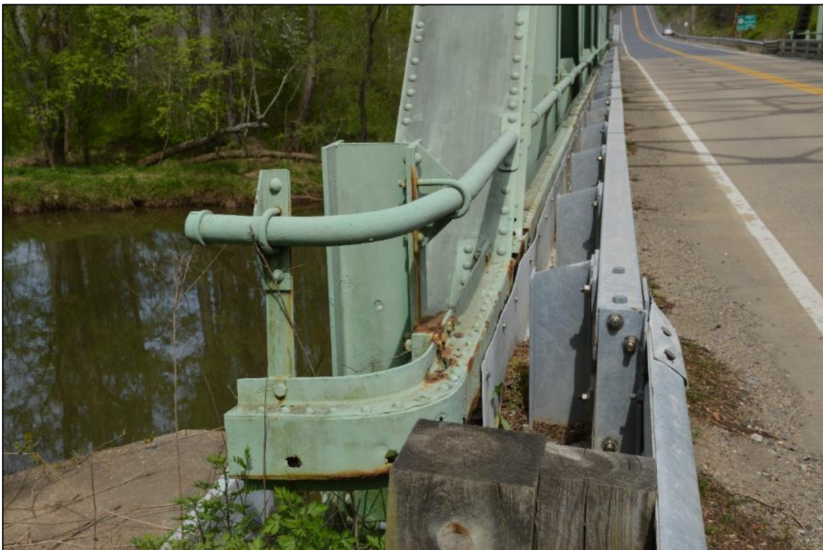
Photo 3: Detail of original handrail and channel at southwest end of upstream truss, view east. Note debris accumulation at base of splash shield.
