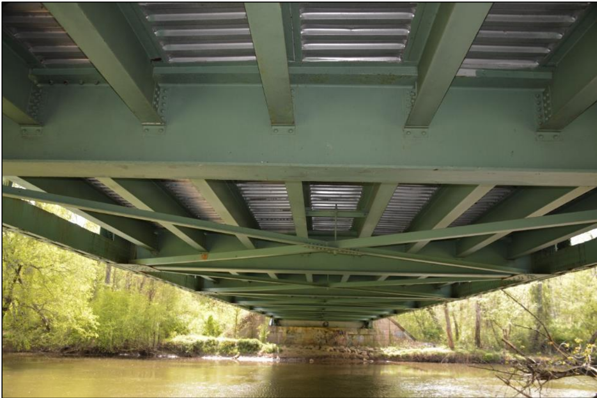
Photo 4: Painted floor system and deck, completed in 2007.
