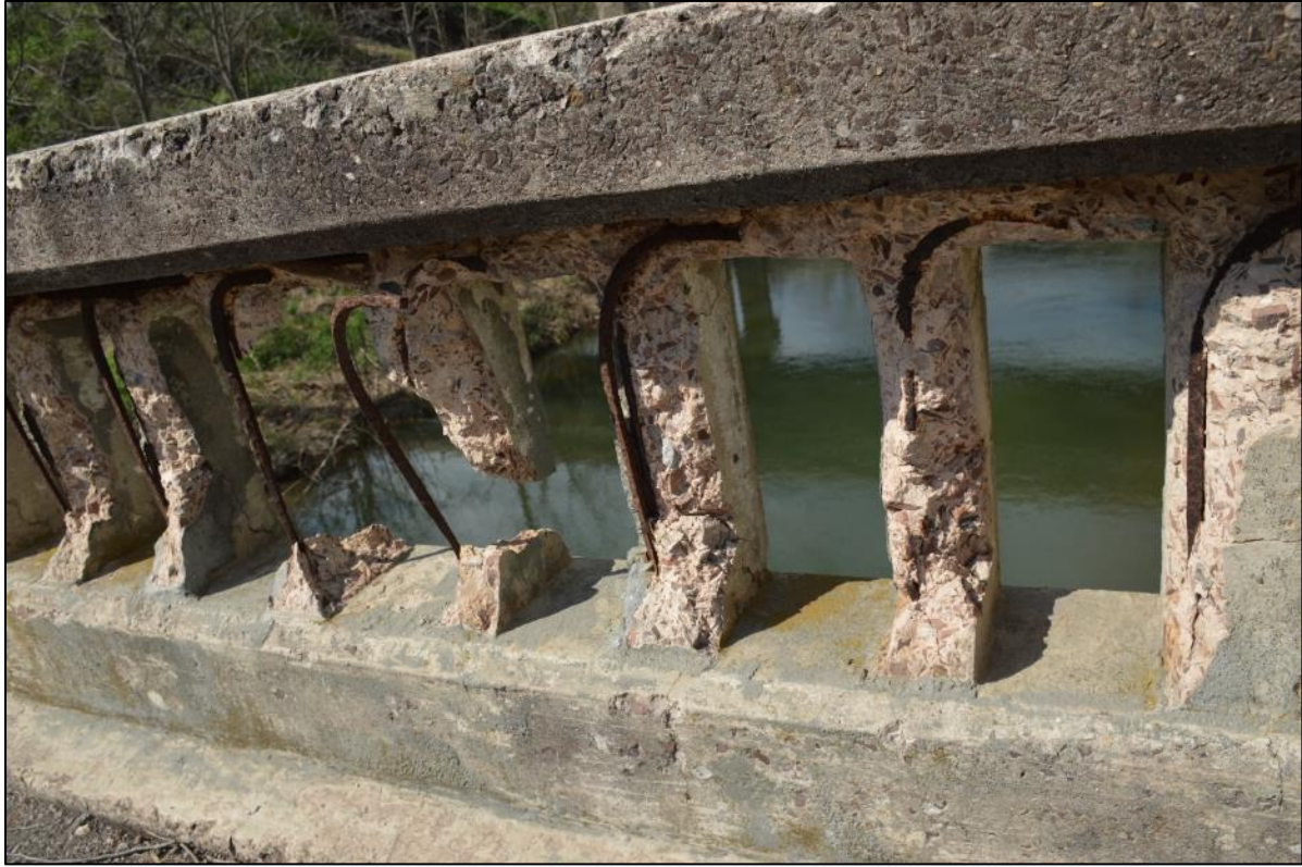
Photo 4: Detail of mortar deterioration and exposed rebar on original balustrade.
