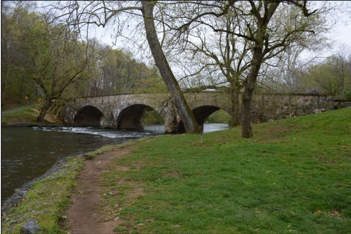
Photo 1: Upstream elevation of bridge, view southwest. Note shoring of southeast parapet wall due to accident damage and overhanging mature trees.
