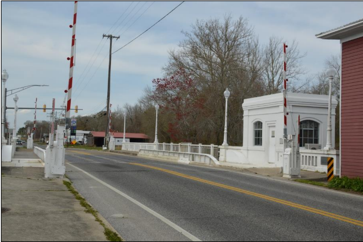
Photo 2: View north of bridge deck, note historic steel railing on bascule span.
