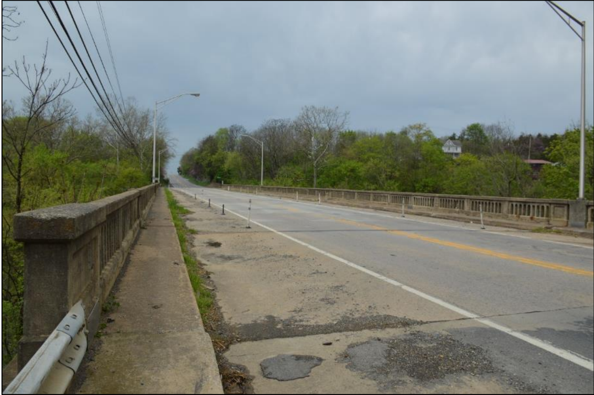
Photo 4: View of deck. Note pedestal and pigeonhole design of original balustrade, sidewalk, and non-historic lighting.
