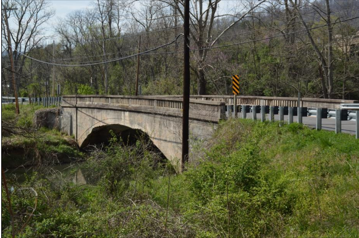
Photo 1: Downstream elevation of bridge. Note PVC drains installed in the southwest and southeast abutments. View northwest.
