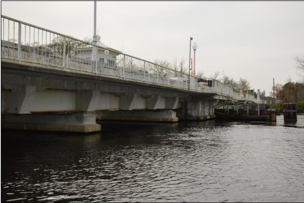
Photo 4: View of replacement steel girder replacement spans, looking southwest.
