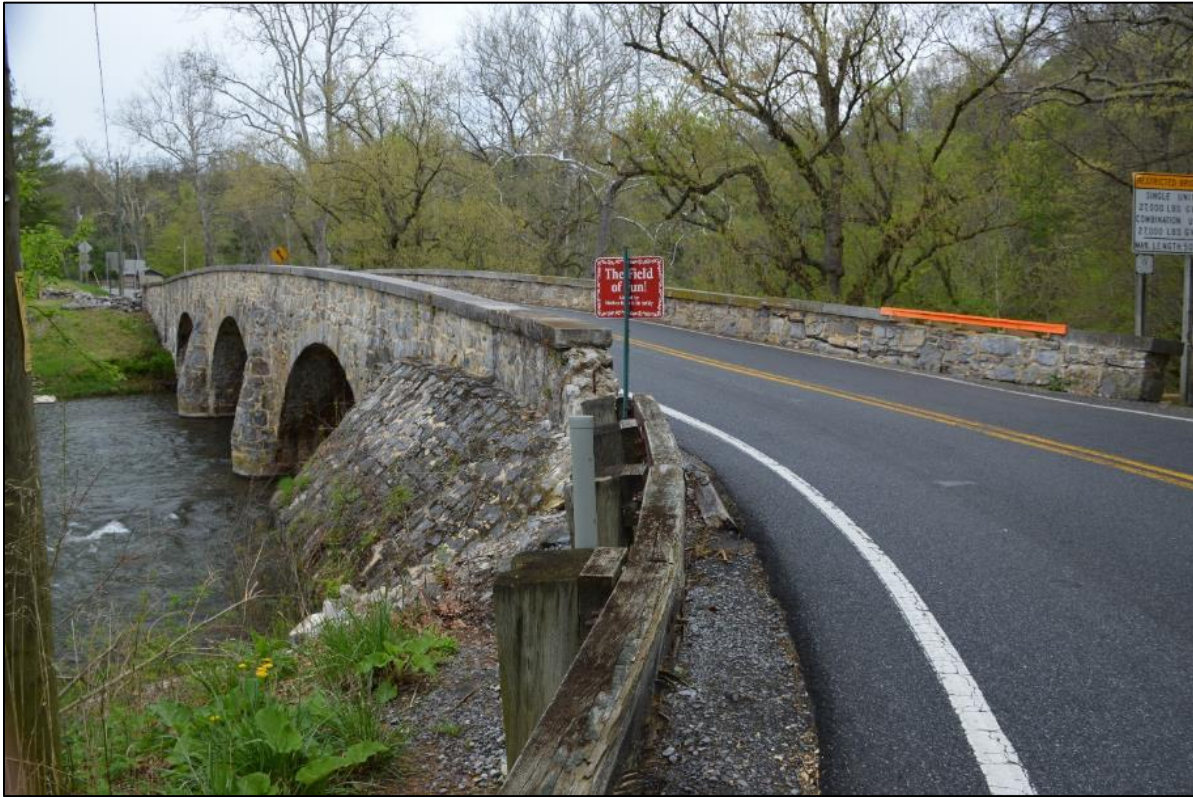
Photo 4: South approach. Both parapets show vehicular damage, view northeast.
