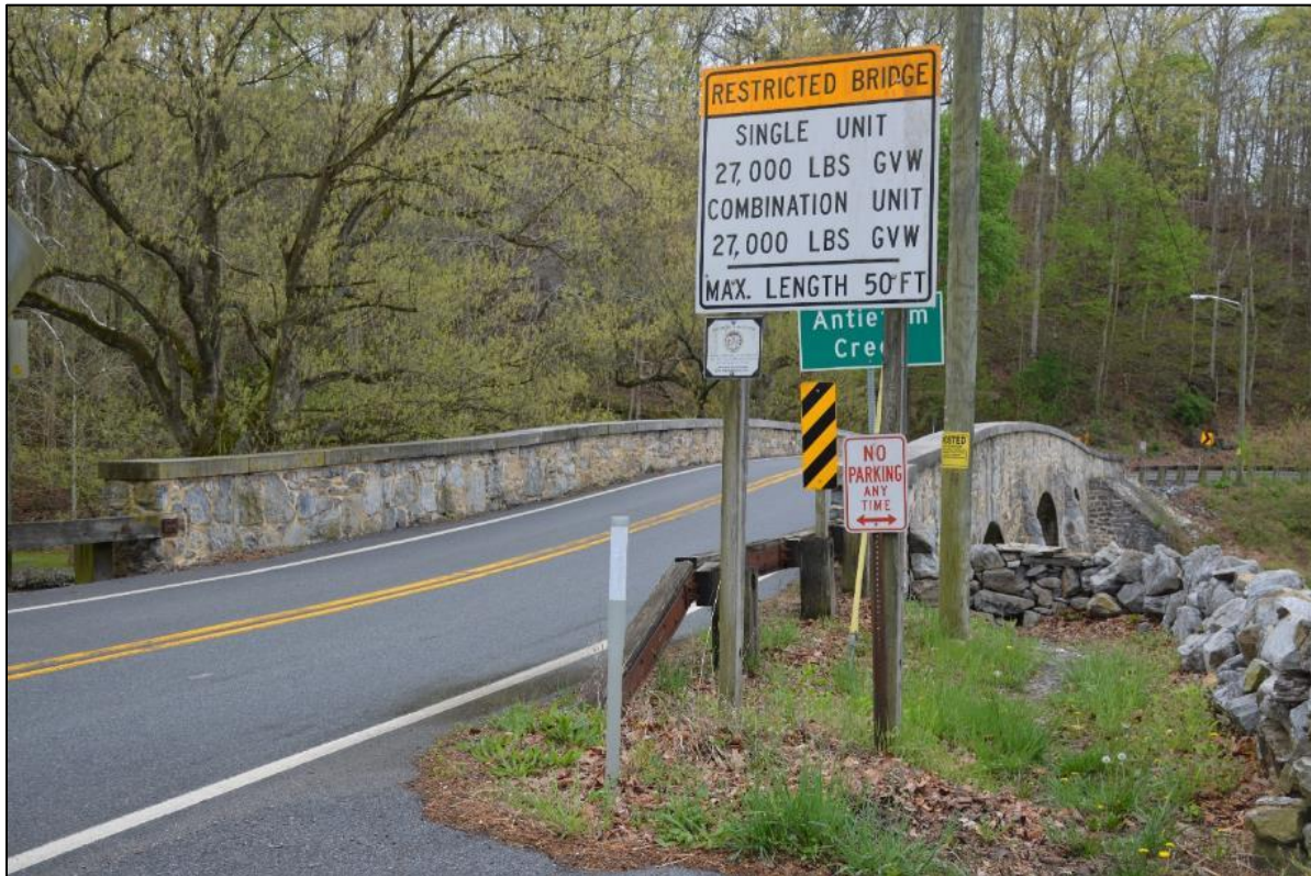
Photo 2: North approach, view southeast. Note context-sensitive steel-backed timber traffic barrier and posted restrictions.
