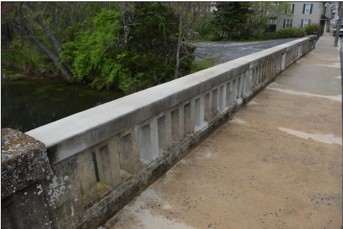
Photo 3: Detail of repaired balustrade, matching the original rectangular openings and railing profile.
