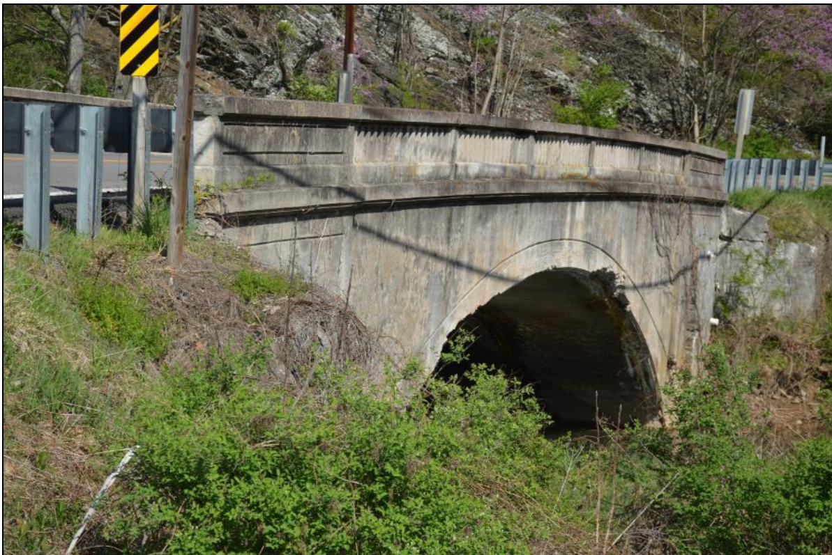
Photo 3: Note failing concrete at barrel of arch, view northeast.
