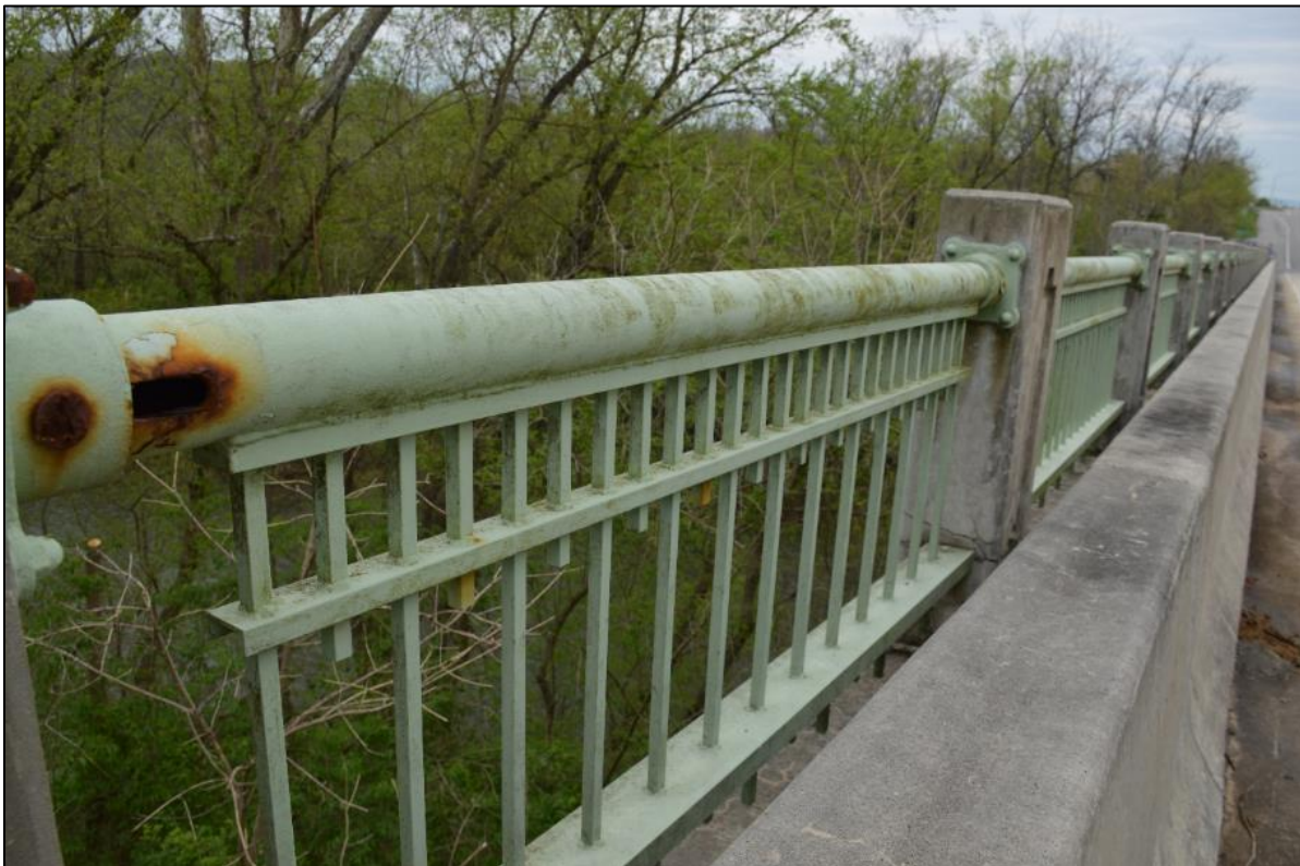
Photo 3: Detail of salvaged railing, replicated pilaster, and safety barrier.
