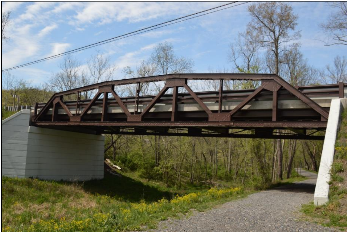
Photo 1: View of bridge from towpath, looking northwest. Note plating in channel of lower chord.
