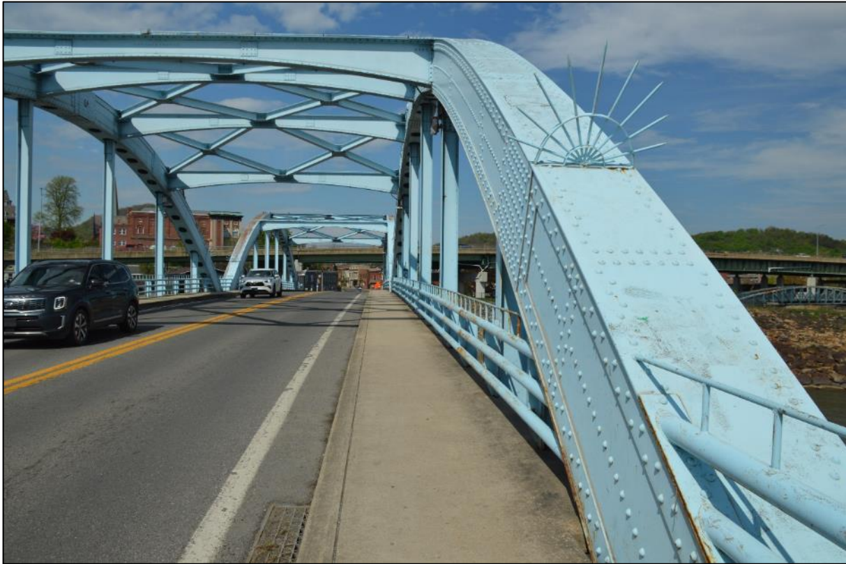
Photo 2: View of bridge deck showing width of traffic lane and sidewalk as well as the original 3-rail railing and top rail extension that are attached to arch and suspenders, view northwest.
