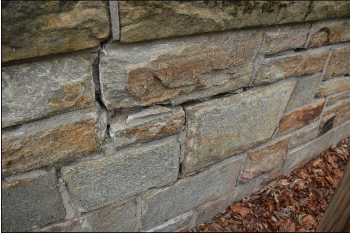
Photo 4: Detail of mortar deterioration on interior face of veneer parapet. Note accumulation of leaf litter.
