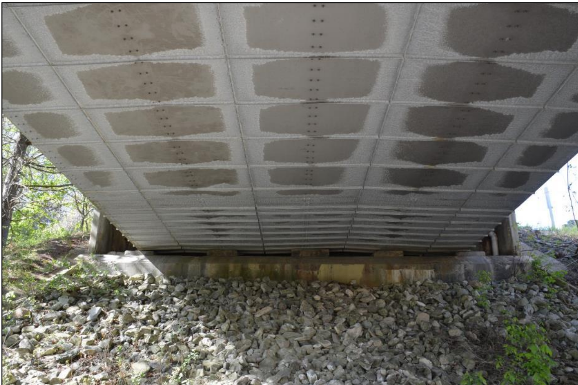
Photo 3: Underside of superstructure, view west. Girder is formed of five connected hollow triangular box beams.
