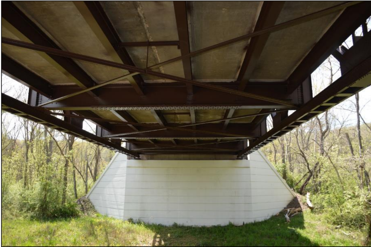
Photo 4: View of repaired abutment from towpath. Additional plating and new rivets visible on floor beam flange, view west.
