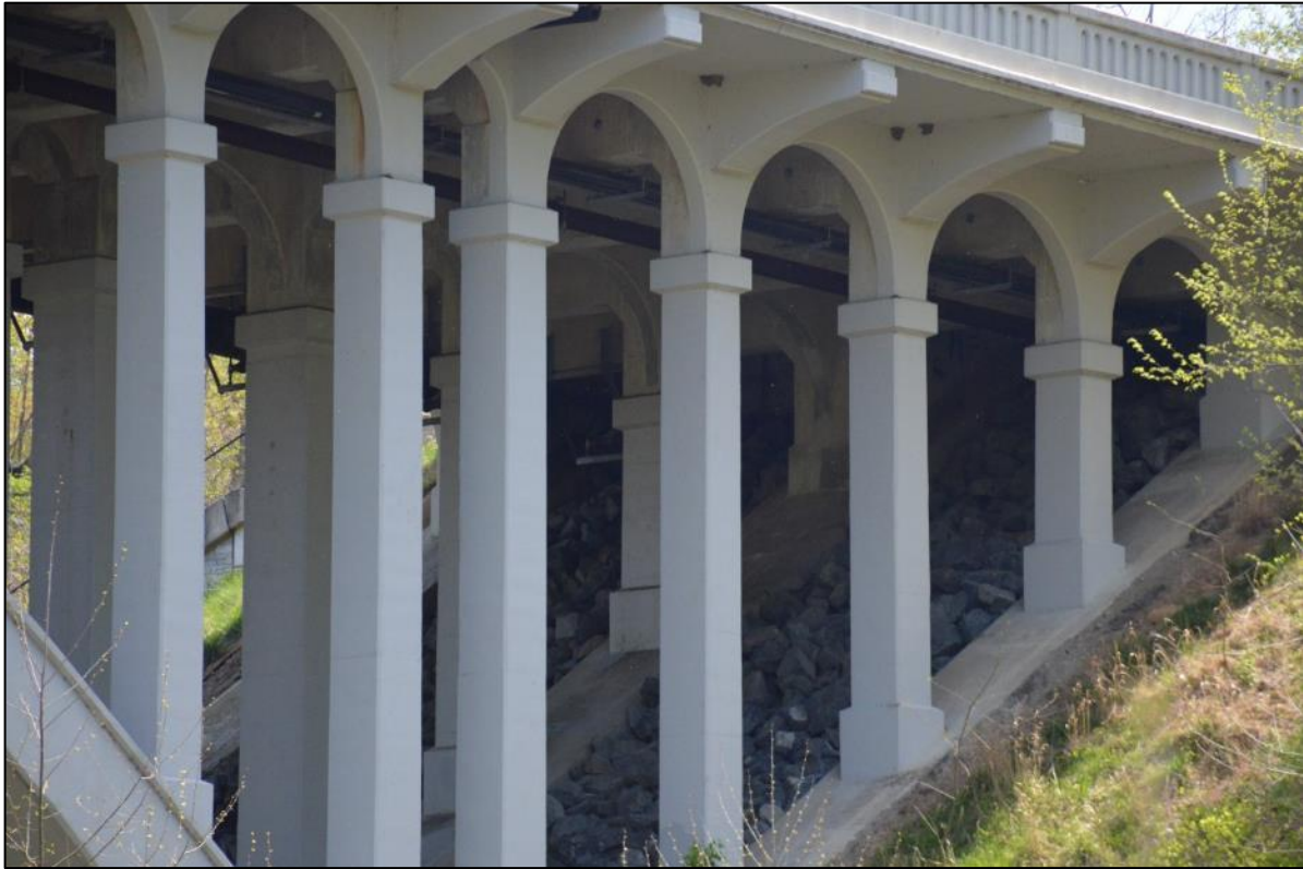
Photo 2: Detail of spandrel columns and brackets supporting new deck. Note indentations in solid safety barrier.
