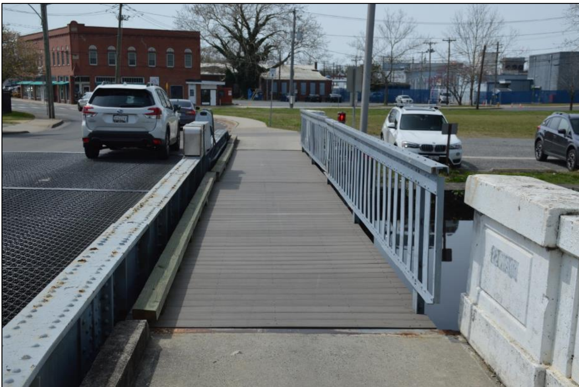
Photo 3: View of timber sidewalk railing, steel deck and bascule girder. View west.
