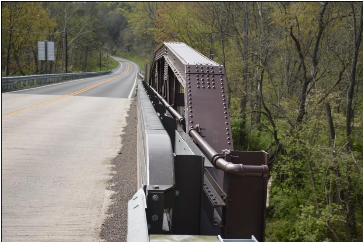
Photo 3: Historic handrail behind fiberglass shield and new 3-rail barrier, view west.
