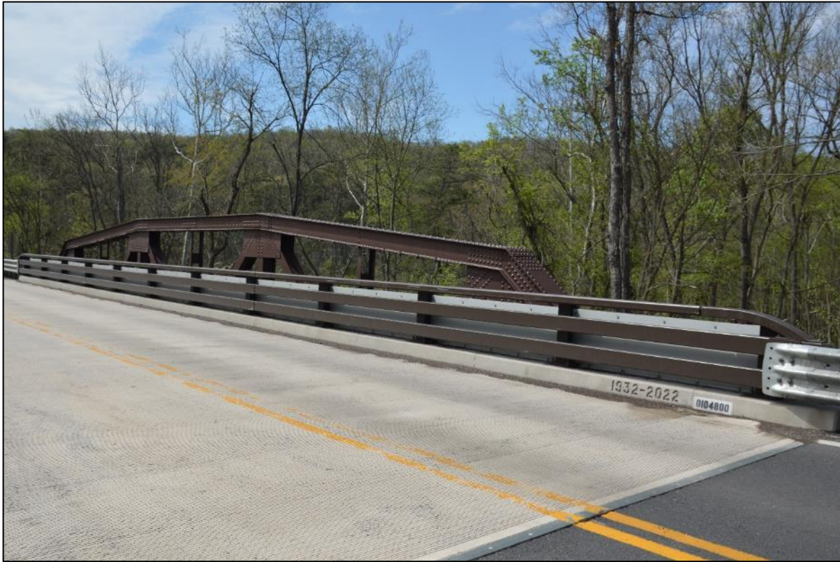
Photo 2: View northwest of 3-rail barrier and fiberglass spray shield. Rehabilitation date at curb.
