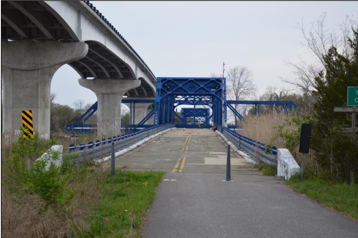
Photo 1: South approach spans and fixed truss span. Note new bridge upstream/left and original railings.
