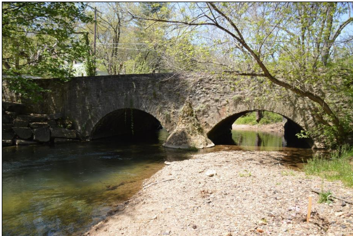
Photo 1: View of east/downstream spandrel walls and pier, view northwest. Note abundance of vegetation.
