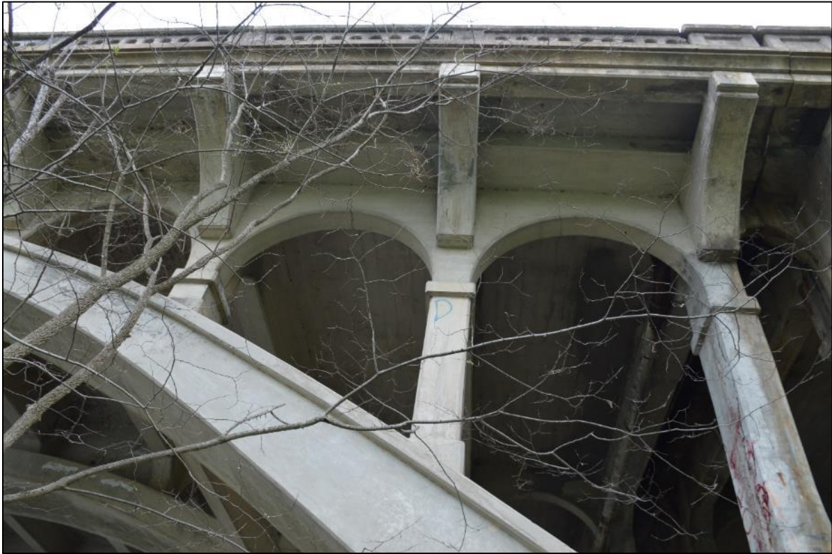
Photo 2: Detail of spandrel columns and brackets supporting sidewalk at east span.
