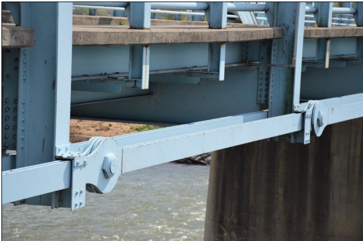
Photo 3: Detail of suspender and hangers.
