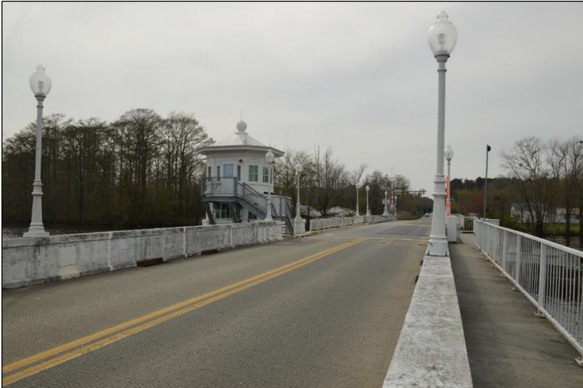
Photo 2: View of bridge deck from eastern approach spans, note replica light fixtures and non-historic steel railing.
