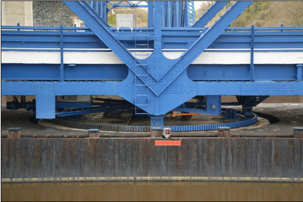
Photo 4: Detail of pivot pier, drum, and pivot mechanism.
