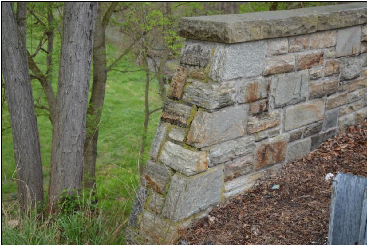
Photo 3: Northwest end of parapet. Note debris accumulation at base and proximity of trees, view north.
