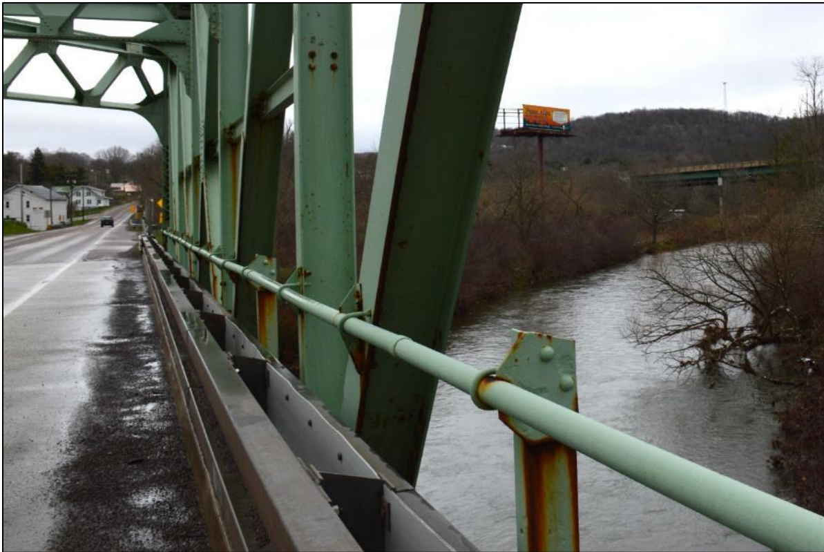
Photo 2: Detail of historic handrail and updated 2-rail railing and fiberglass shield to left, view east. Note deposition of material at curb.
