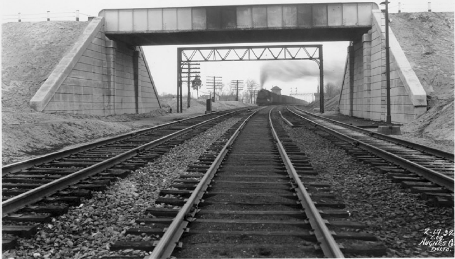
PLATE 10: : Typical Metal Plate Girder (Through) Bridge: Crossing Railroad Tracks at Severn
