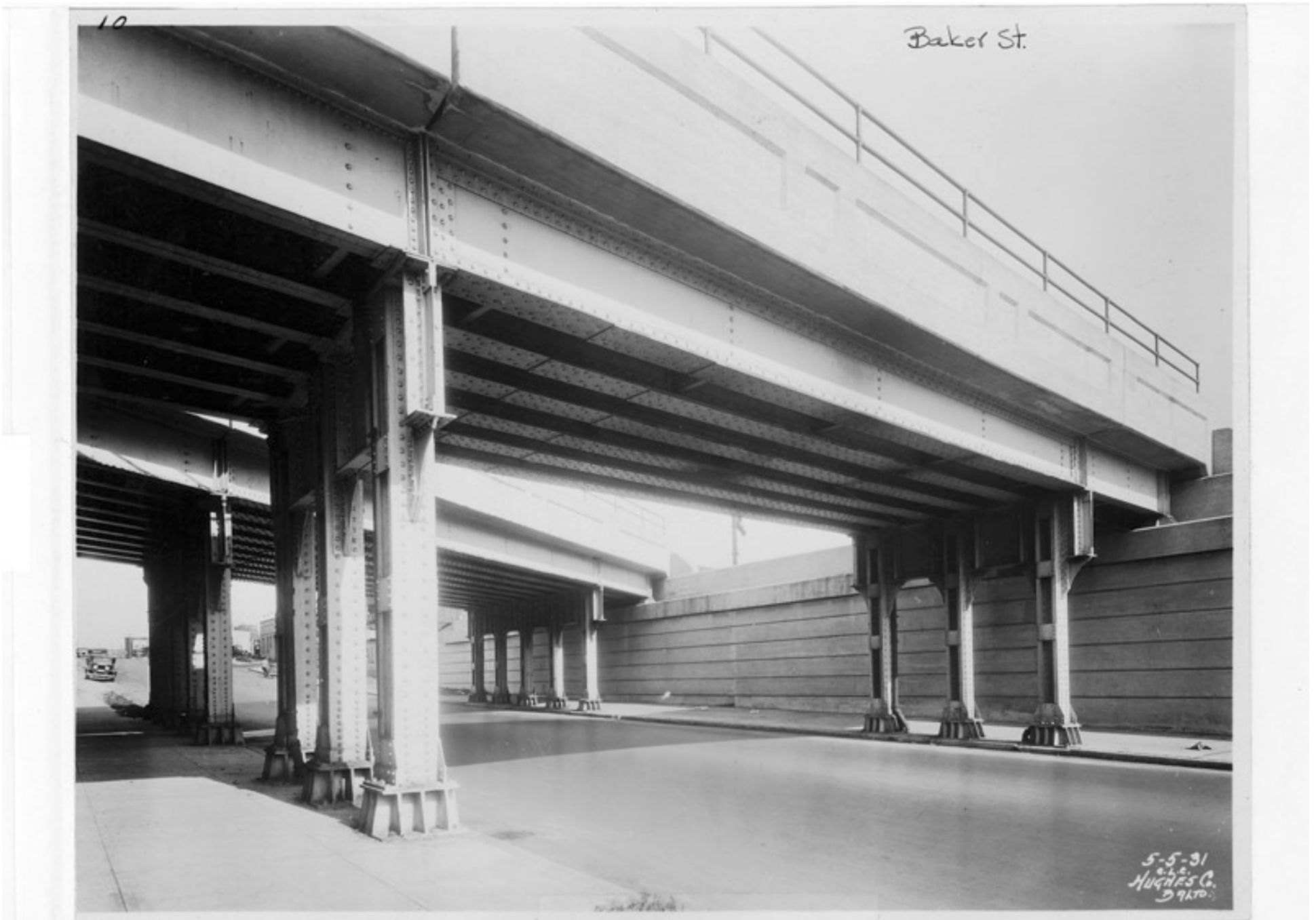
PLATE 11: Typical Metal Plate Girder (Deck) Bridge: Bridge on Baker Street in Baltimore
