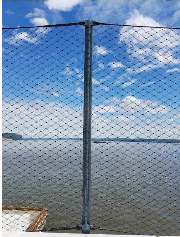
Figure C4. Tappan Zee Bridge
