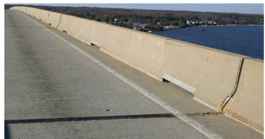
Figure 2. Existing Bridge Parapet
