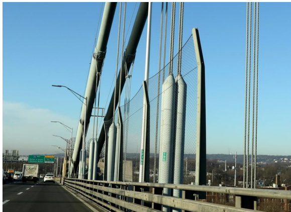
Figure C2. Verrazano Narrows Bridge
