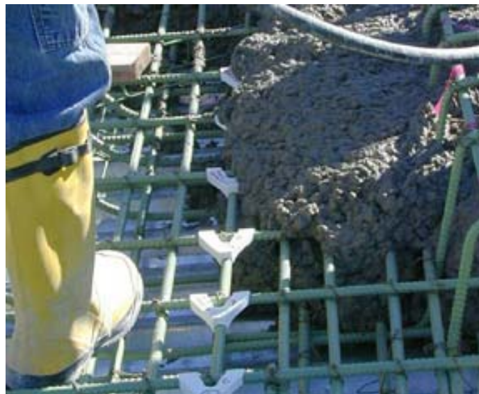
Figure 15 - Bridge Installation of Smart Aggregate in holders
