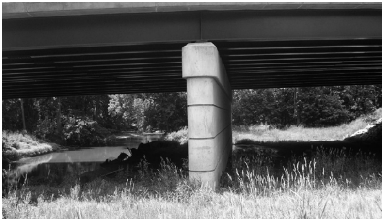
Figure 3.2. MD 355 over Great Seneca Creek (existing bridge).
