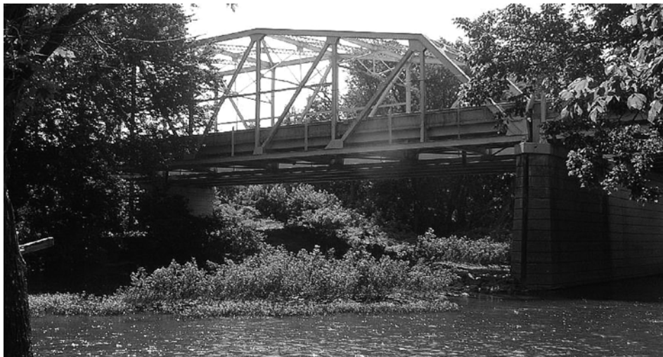
Figure 3.3. MD 26 over Monocacy River (existing bridge).
