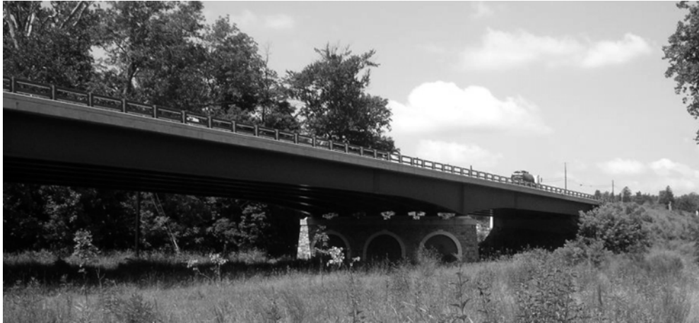
Figure 3.1. MD 28 over Seneca Creek (existing bridge).
