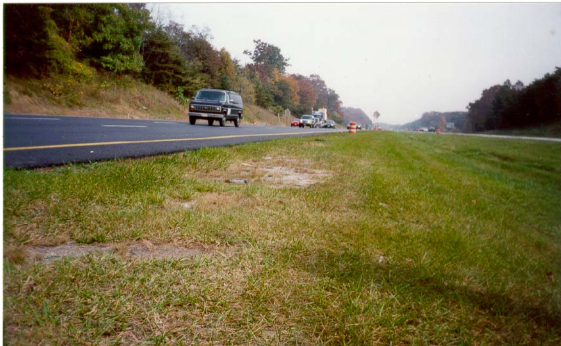
Photograph 2: Patchy grass growing in the median strip on I-70 after approximately one year.
