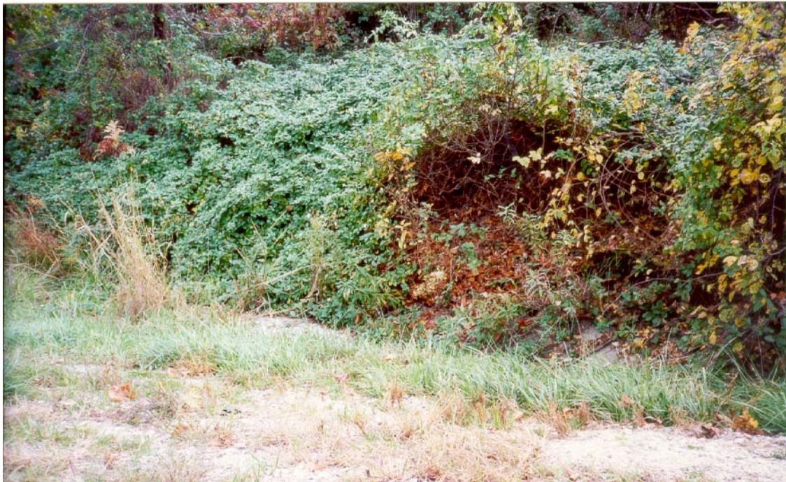
Photograph 4. A view of the road shoulder designed by SHA 50/50 soil/gravel mixture
