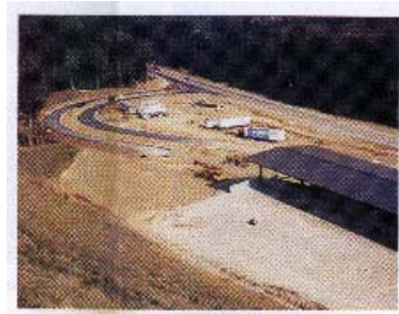
Photograph 3. The fully stabilized slope after construction (Presto Products Co., 1998).
