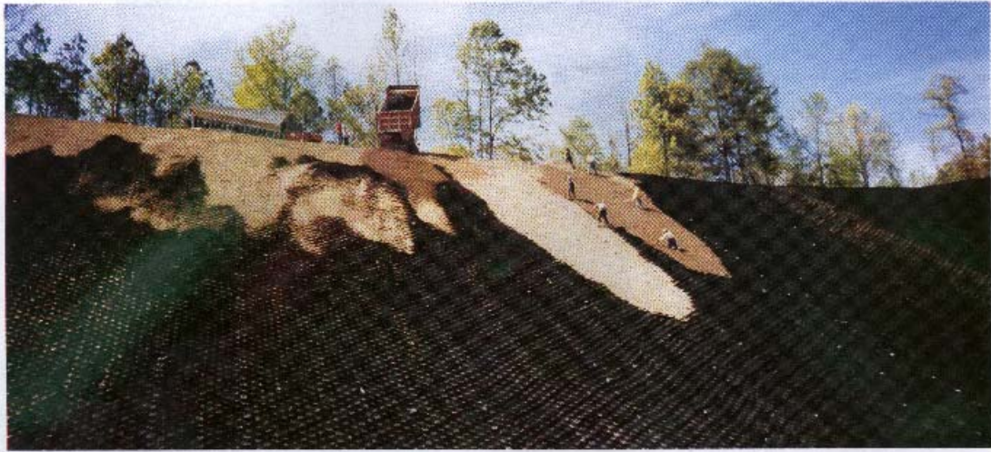
Photograph 2. Infill is spread over the cellular-confinement system as installers rake the materials into the cells (Presto Products Co., 1998).
