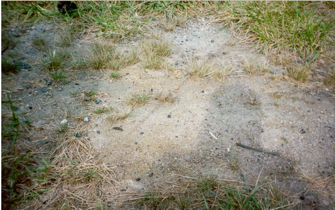
Photograph 3: The SHA's attempt at vegetating the shoulder backfill using a 50/50 soil/gravel mixture
