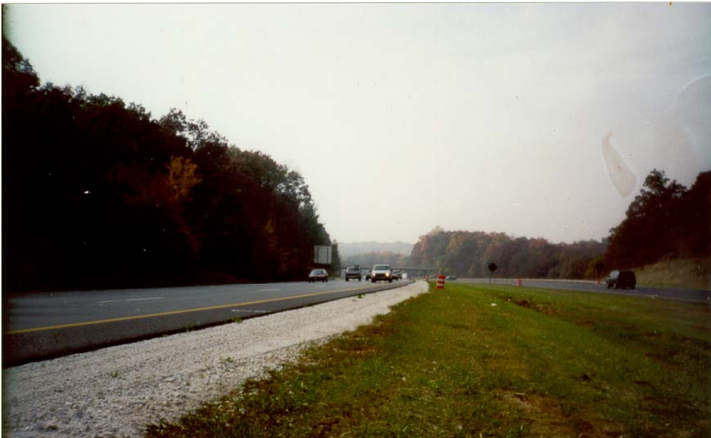
Photograph 6. This is a picture taken from I-70, near Columbia, Maryland; this shows the interface between the road shoulder and the vegetated median in the middle.
