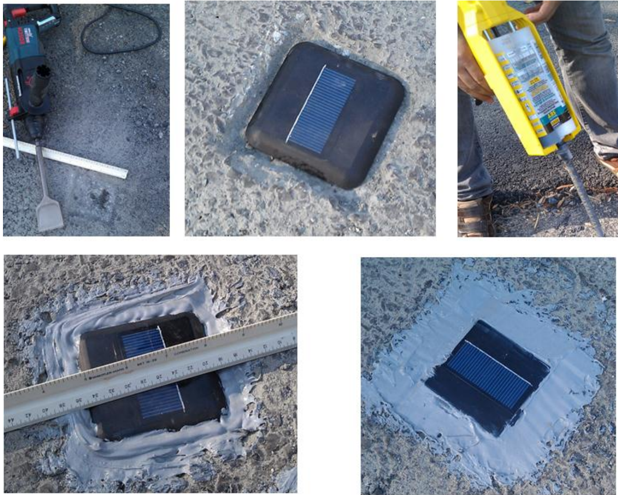
Figure 18. Testing adhesive and testing installation steps for freeway deployment
