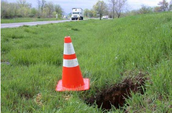
**Figure 18. Incipient sinkhole in unlined roadside drainage in the median of Interstate 81.**
