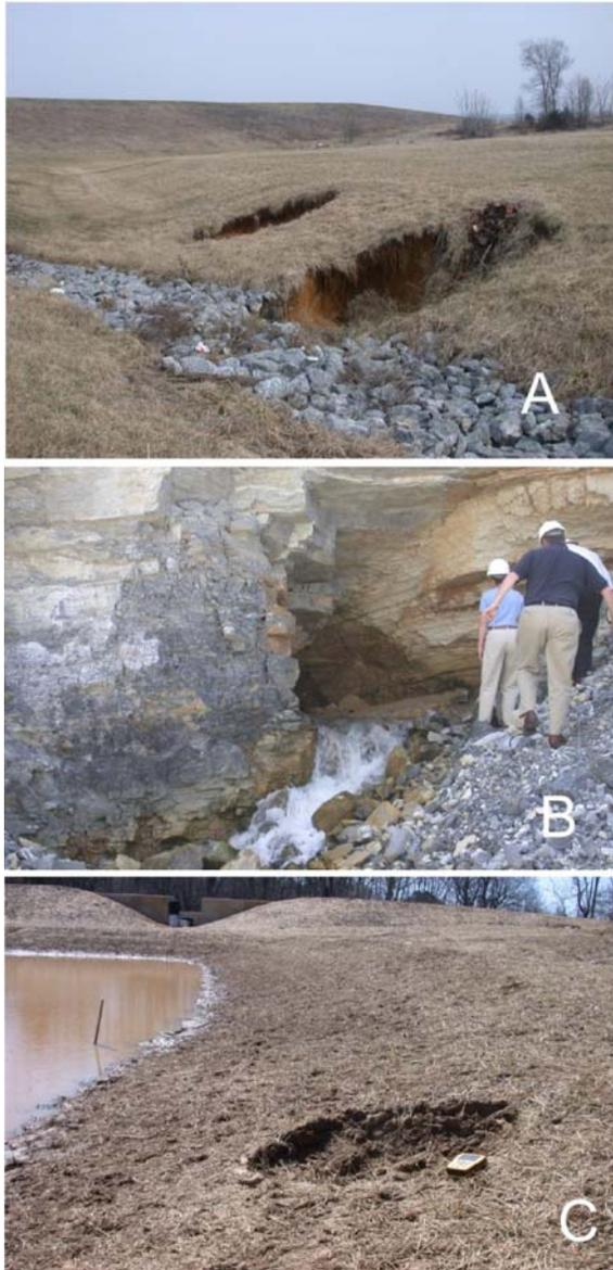
**Figure 16. Some human-induced karst problems. A. Unlined drain within the Rockdale Run Formation at Hagerstown Airport producing sinkhole activity. B. Opening of cave in Conococheague Formation by quarrying in eastern Hagerstown. C. Sinkhole activity in newly created storm water management pond.**
