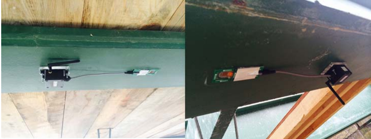
Figure 14: Wireless strain sensors deployed in Span 2 and Span 3 of the bridge.
