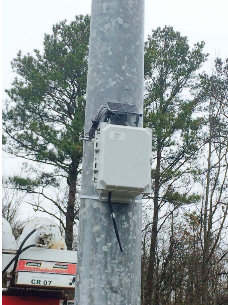
Figure 15: Solar powered wireless cellular gateway.
