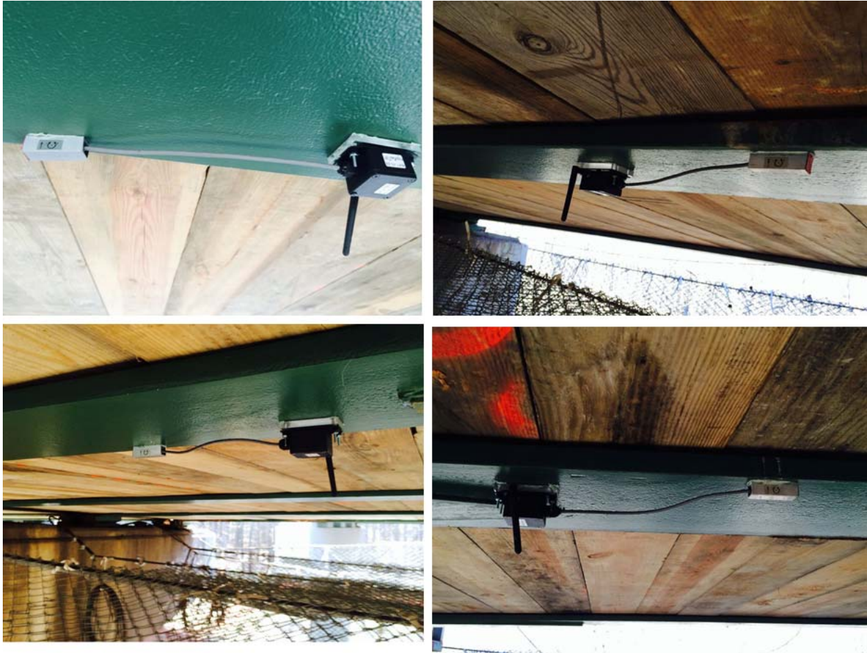
Figure 13: Sample pictures of wireless inclinometer sensors deployed in Span 2 and Span 3 of the bridge.
