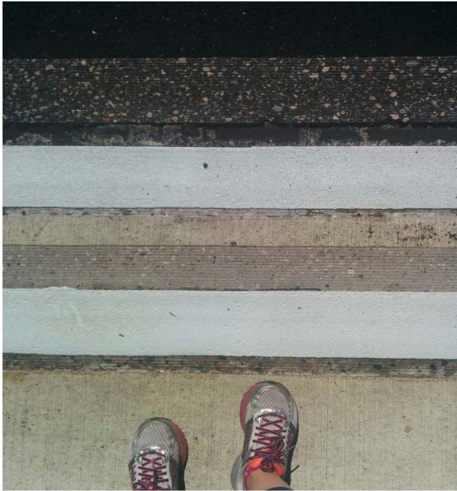
**Figure 6-2 Detail A: Ground-in/In-line cycle rumble strip**
