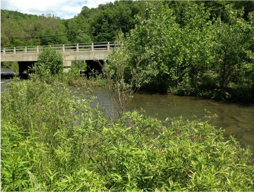
Figure 9. MD 36 over Georges Creek standing upstream on lowered flood plain showing aggradation and woody vegetation accumulating in right span.
