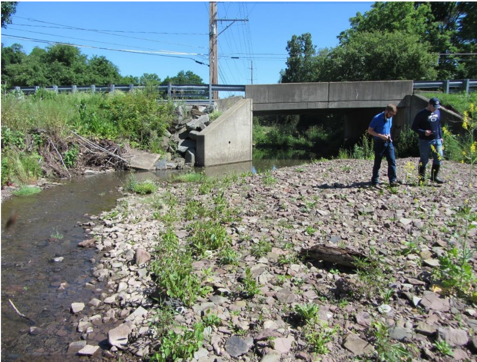
Figure 4. PA 3036 over S. Branch Sugar Creek near Troy, PA.
