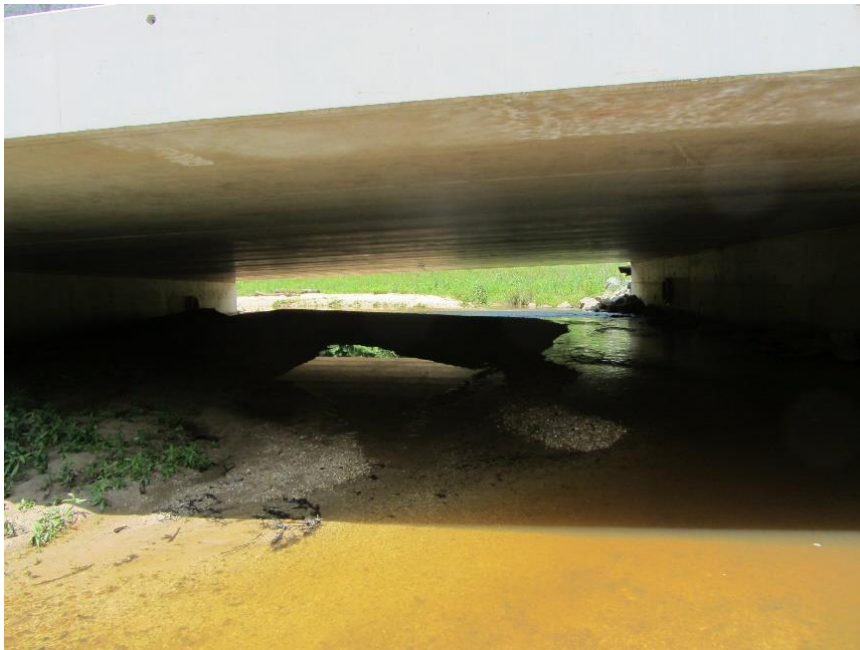
Figure 13b. Looking upstream under the bridge. Note the deposition in the left of the picture.
