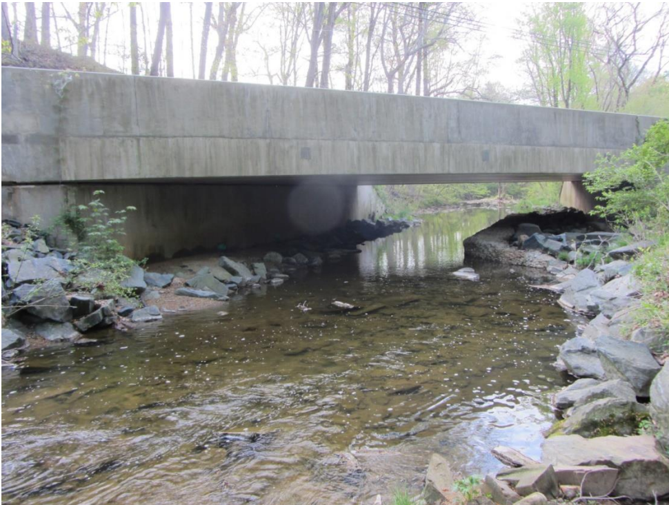
Figure 19. MD 136 over Broad Run looking downstream at the bridge opening. The previous bridge abutments were left under the reconstructed bridge.
