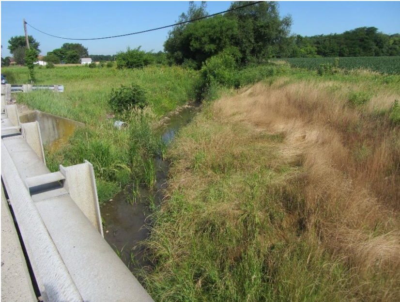
Figure 5b. Post construction.
