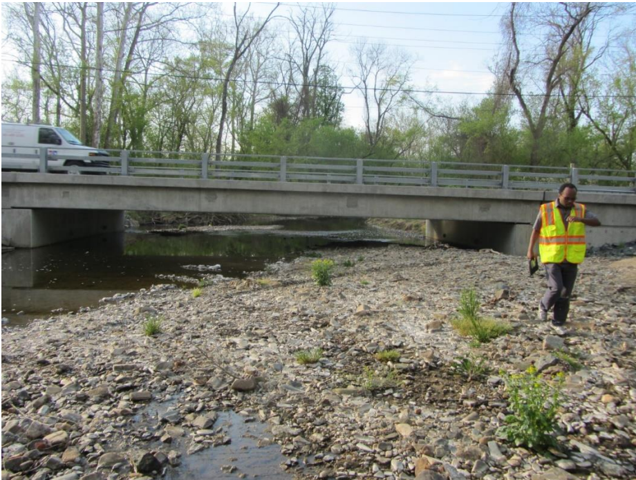
Figure 21. Looking downstream at MD 7 over James Run. Sediment accumulation on the right bar appears to be moving downstream through the bridge opening.
