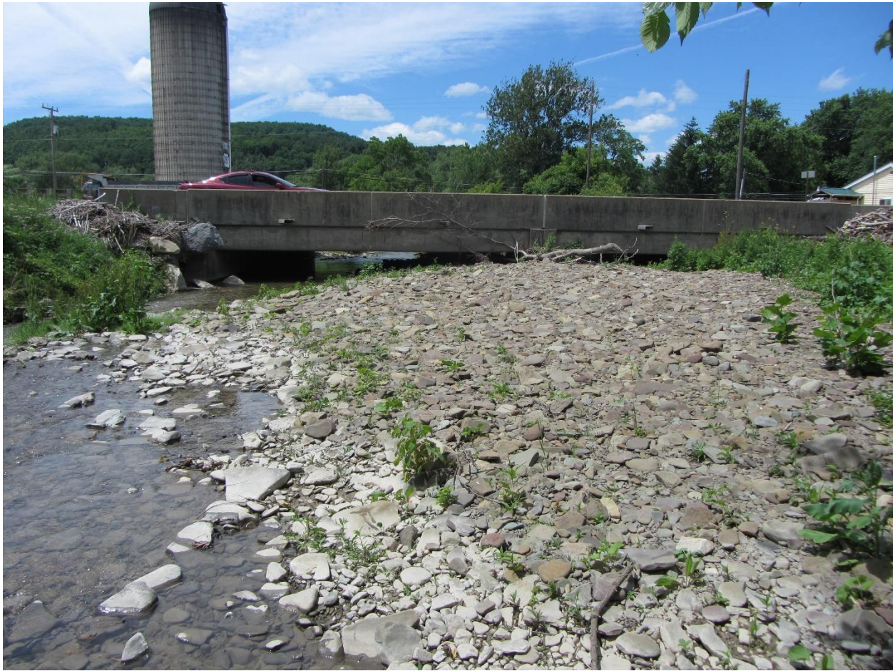
Figure 6. Severe sediment deposition at PA 287 over Mitchell Creek, north of Tioga, PA.
