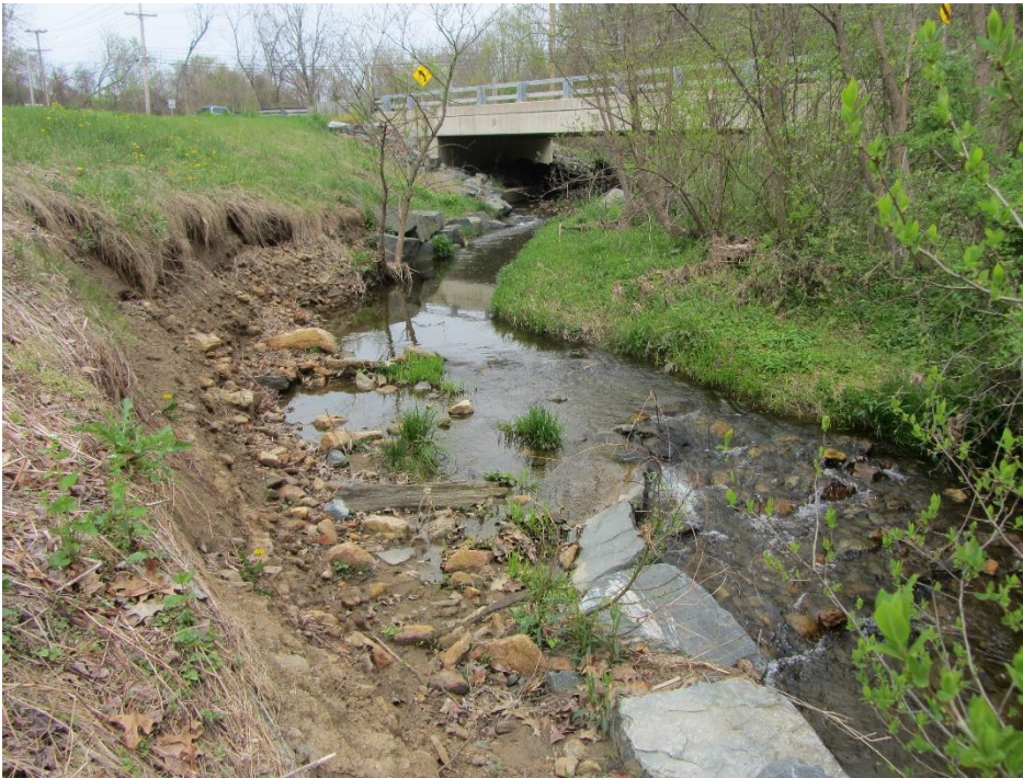
Figure 17. Downstream of MD 165 over tributary to the West Branch of Winters Run, facing upstream. Vanes in the channel have failed to control bank erosion on the right bank.
