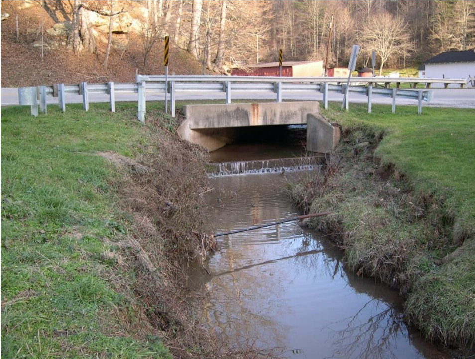
Figure 3. Stream channel degradation. U.S. Rt. 199 N, 0.8 km S of Gandeville, WV.
