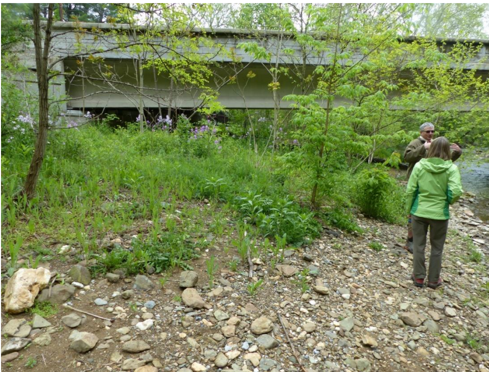
Figure 10. MD 17 over Middle Creek standing upstream looking downstream showing aggradation occurring on left bank.
