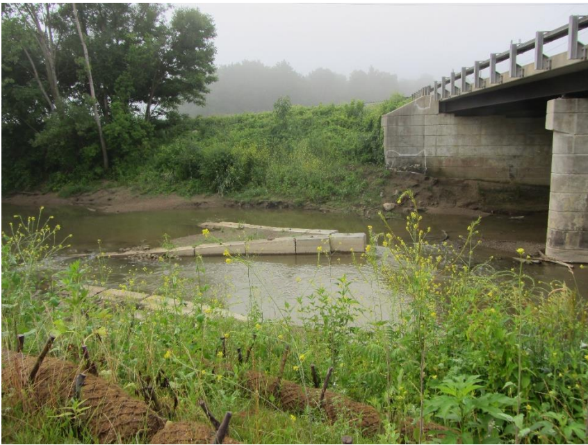
Figure 7b. Partial w-weir installed upstream of the bridge in Fall, 2015.
