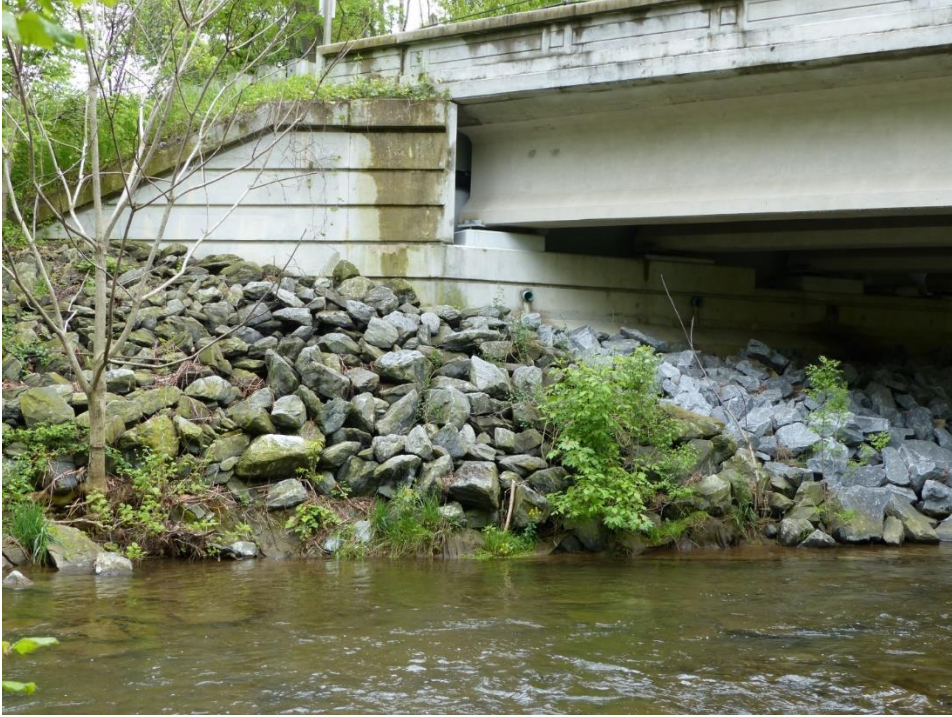
Figure 11. MD 17 over Middle Creek. Undermining of Riprap on downstream right bank.
