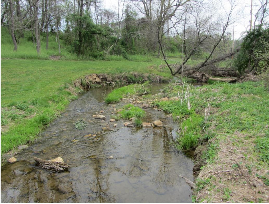
Figure 16. MD 165 over tributary to the West Branch of Winters Run, facing downstream toward the bridge. Note the lateral erosion, poorly functioning vanes, and woody debris in the channel.
