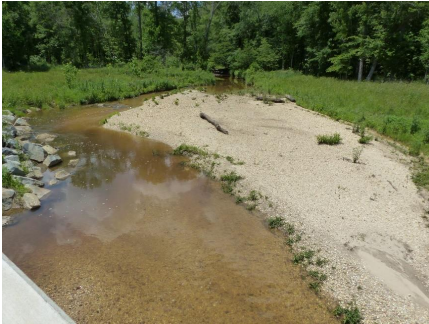
Figure 13a. Bar upstream of the bridge.
