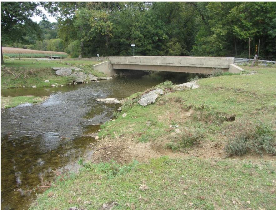
Figure 1b. Looking downstream at bridge.
