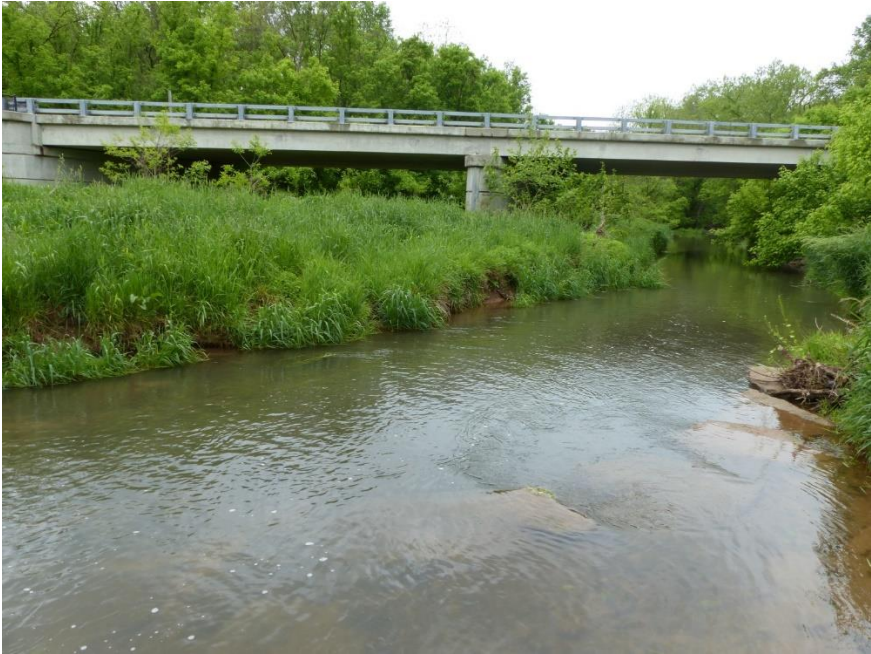
Figure 12. MD 28 standing upstream showing aggradation in left span and rock vane in bottom right of picture.
