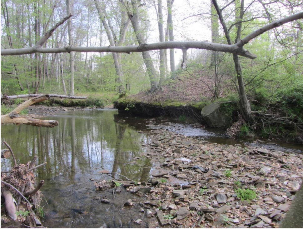
Figure 18. MD 136 over Broad Run, looking upstream from bridge.
