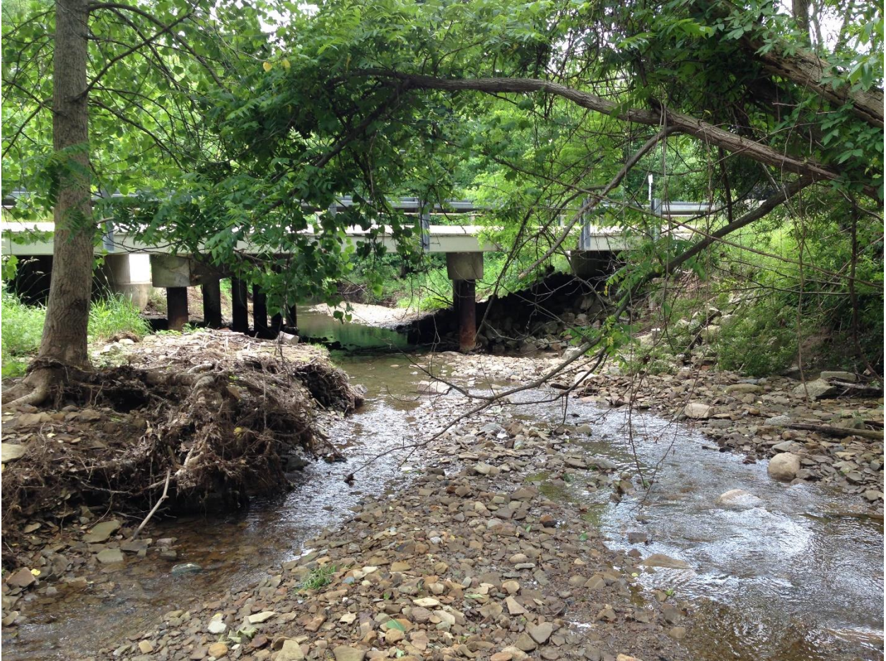
Figure 2. Looking downstream at the Hinckley Hills Road bridge over East Branch of Rocky River in Medina County, Ohio.
