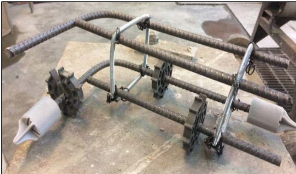
Figure 10: Reinforcement cage for the L-shaped halves
