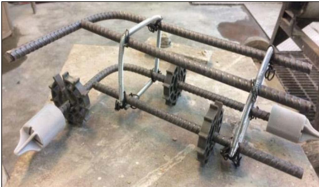
*Figure 10: Reinforcement cage for the L-shaped halves*
