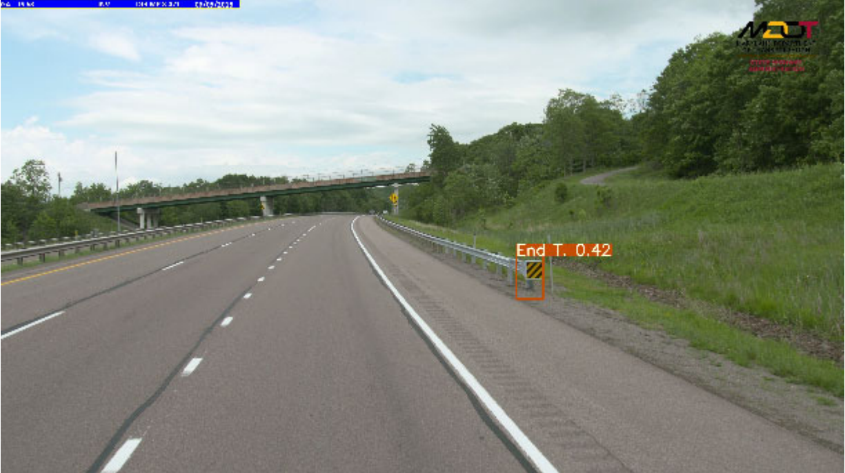
Figure 32. Sample output image with traffic barrier end treatment identified by YOLO v3 model with a bridge in the background
