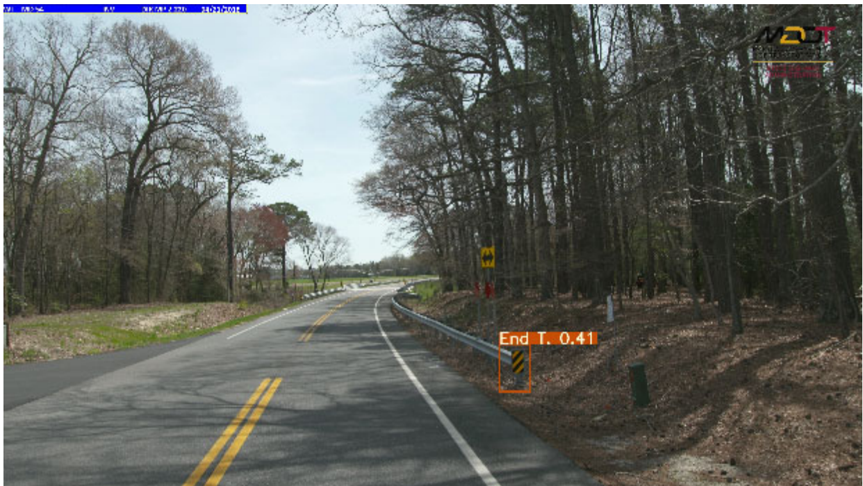
Figure 27. Sample output image with traffic barrier end treatment object identified by YOLO v3 model with medium-scaled traffic barrier end treatment in the picture
