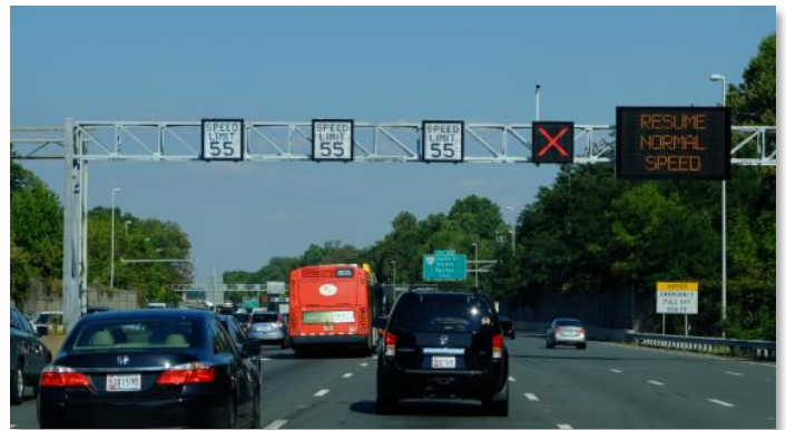
I-66 ATM System designed by WSP
