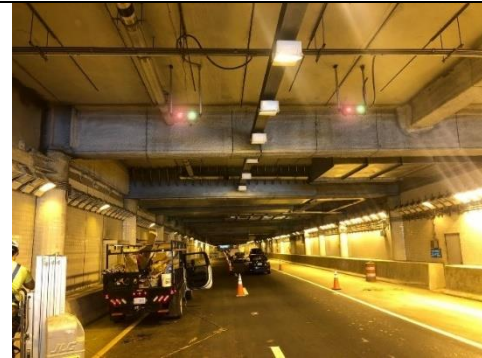
Installing a new design-built system to control Lane Use System lights
