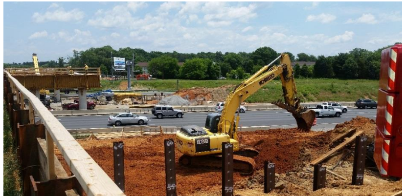
Fall Hill Avenue I-95 Overpass – Phase 1 bridge construction
