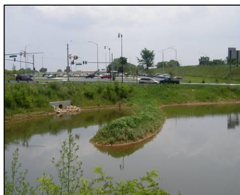
Baffle Constructed from Fill
