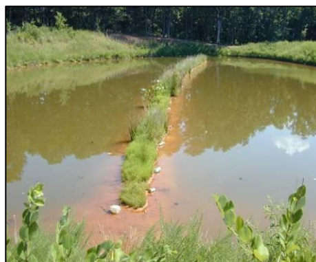
Baffle Constructed from fill eroded after one year
