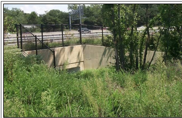
Figure 5-5. Chain Link Railing at Endwall
