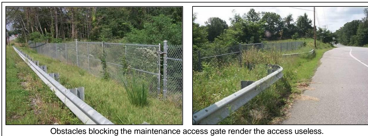
Figure 6-1. Obstructed Maintenance Access
