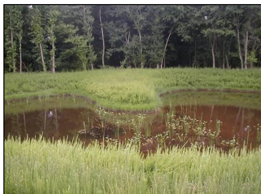
Baffle Constructed In-Situ Holds Form Over Time
