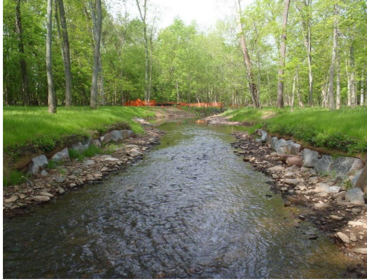
A completed stream restoration project using riffle grade control with stone toe protection
