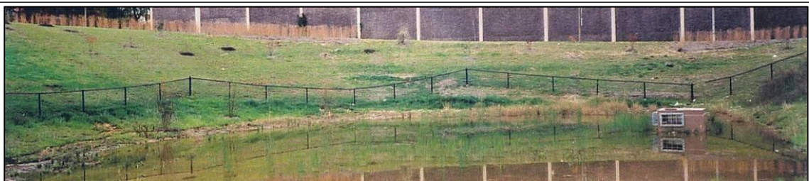
Fence Steps Up and Down Contours (Avoid)
