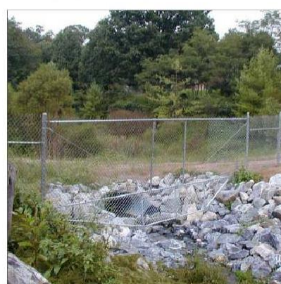
Ditches should be spanned so that debris can flow under the fence, as shown above.
