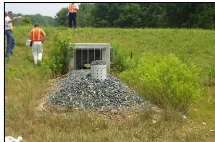
Low Flow Device runs perpendicular to structure (Avoid)
