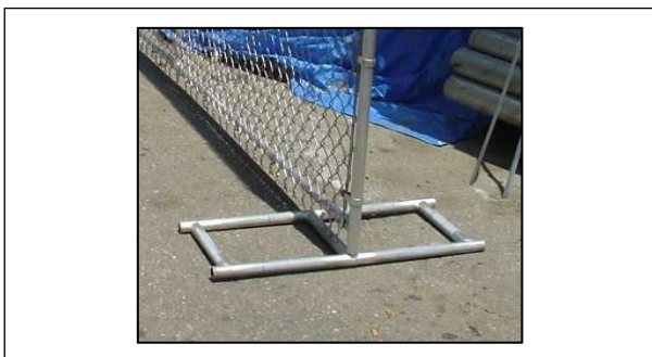
Figure 5-4. Footer at Temporary Fencing
