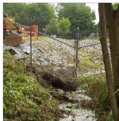
Fencing ditches can be a problem. Refrain from placing the post at the invert of the ditch as shown above. (See photo below)
