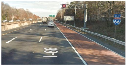
Figure 1 - I-66 Hard Shoulder Running during off-peak Source – Virginia Department of Transportation
