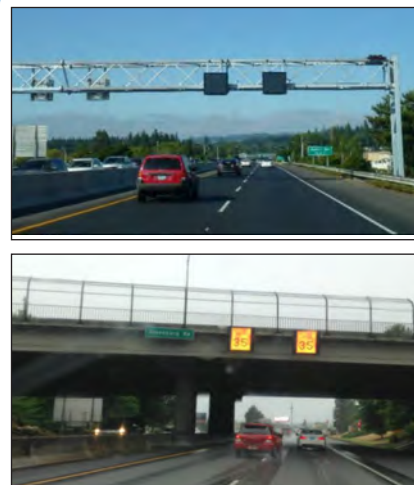
Figure 15: Two Examples of VSL Installations on OR-217
