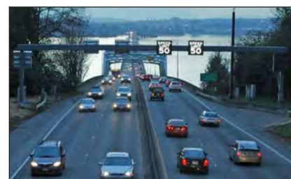
Figure 18: VSL Signs on SR 520, Seattle, Washington
