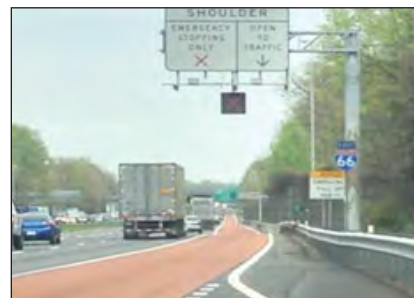
Single Character Overhead Message Sign.
