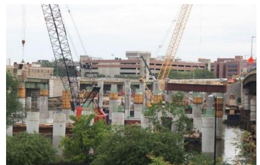
Materials, means and methods used to drive piles within the Anacostia River (11 th Street Corridor) did not generate significant underwater sound waves and vibrations.
