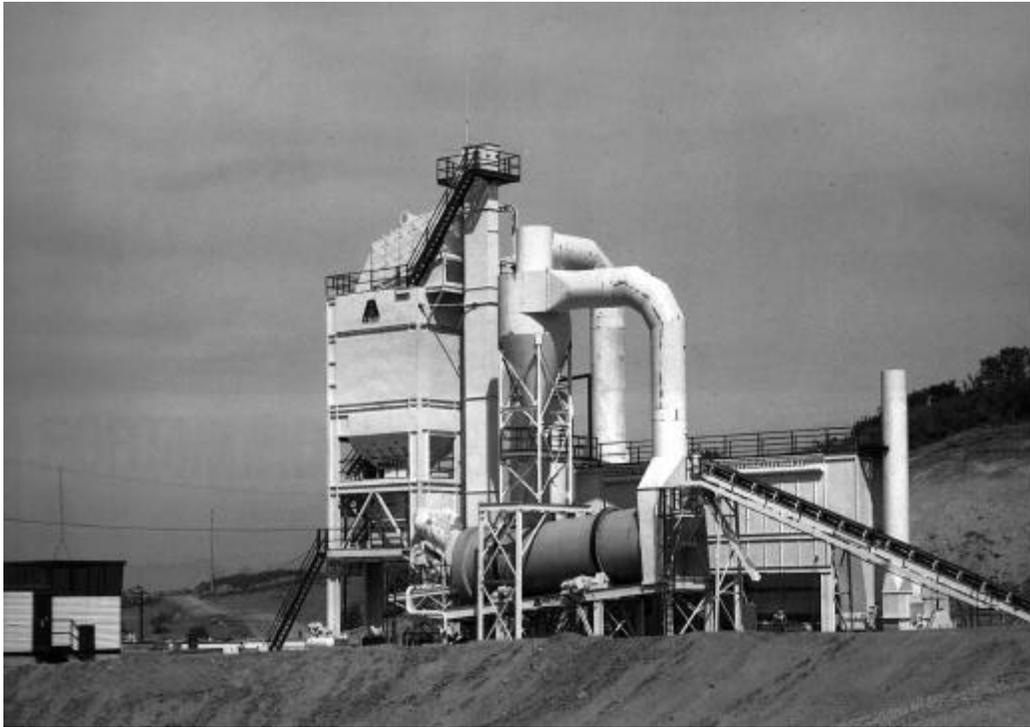
Figure 2.5 Modern HMA batch facility.
