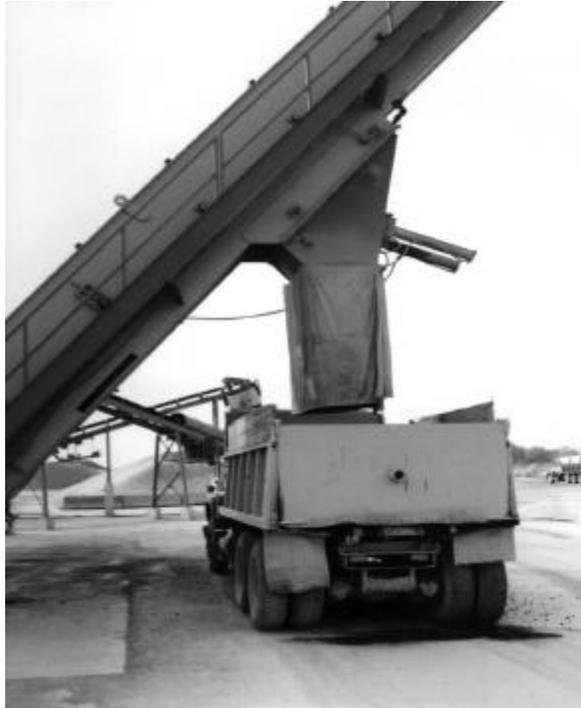
Figure 5.58 "Chop gate" or "drop gate" in slat conveyor.
