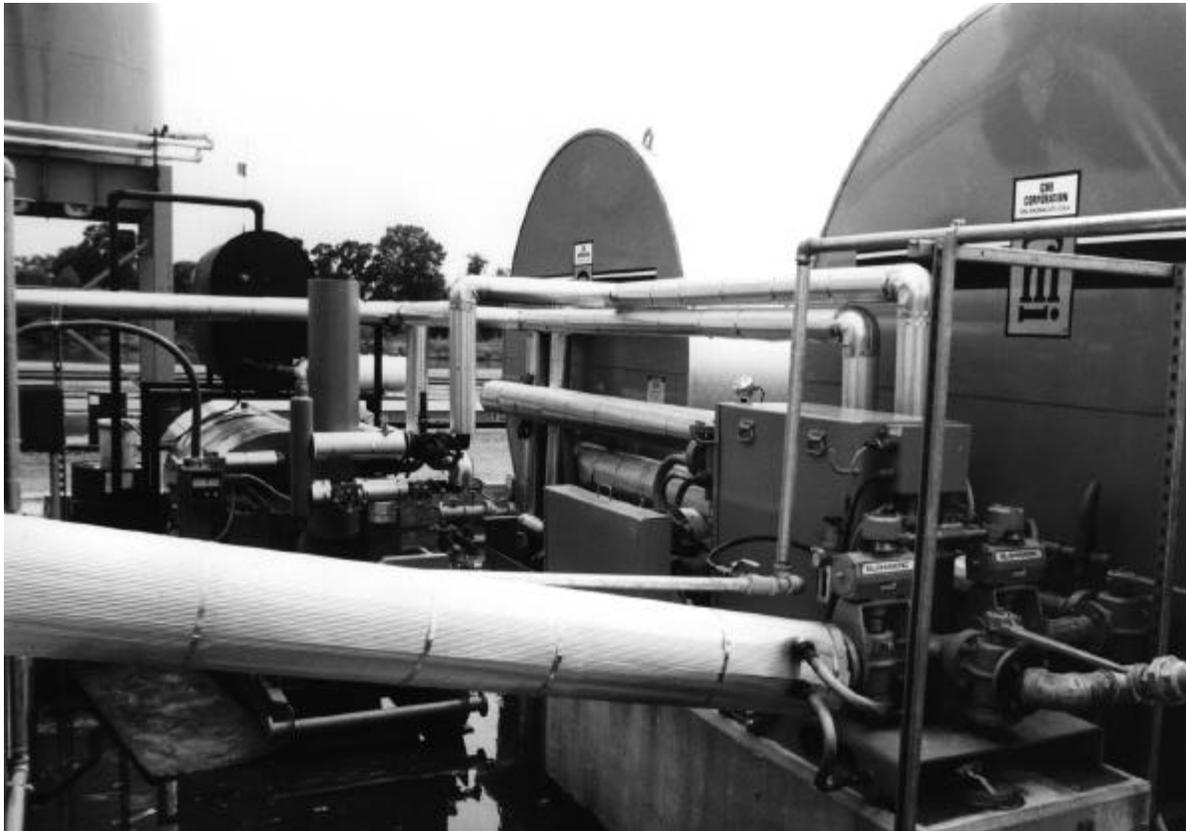
Figure 4.4 Hot oil pipes for asphalt tanks.
