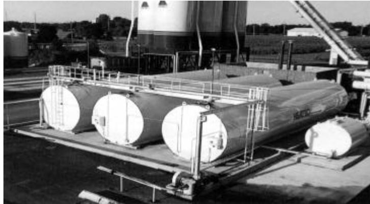
Figure 4.19 Multiple tank installation with transfer lines and heat jacketed valves.
