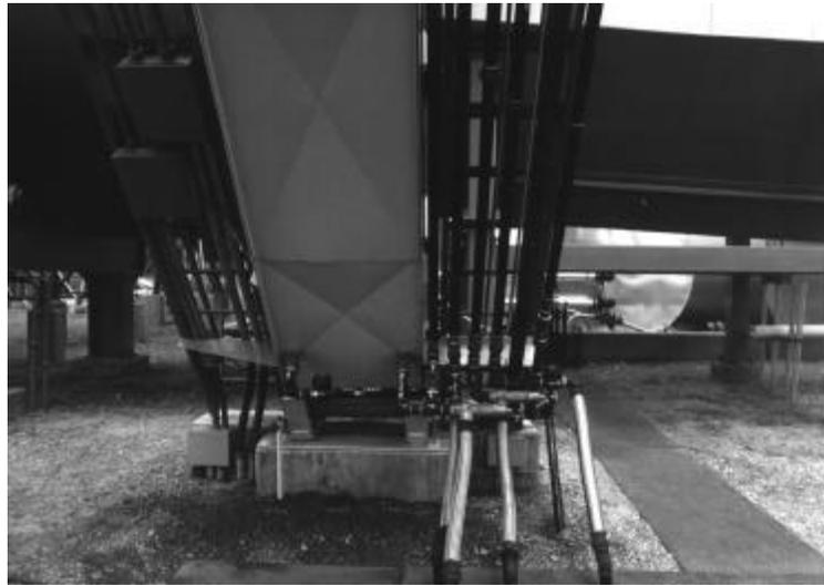
Figure 4.7 Hot oil piping to heat hot mix storage silos.
