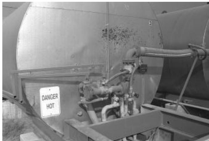
Figure 4.20 Heat jacketed valve with hot oil lines attached.
