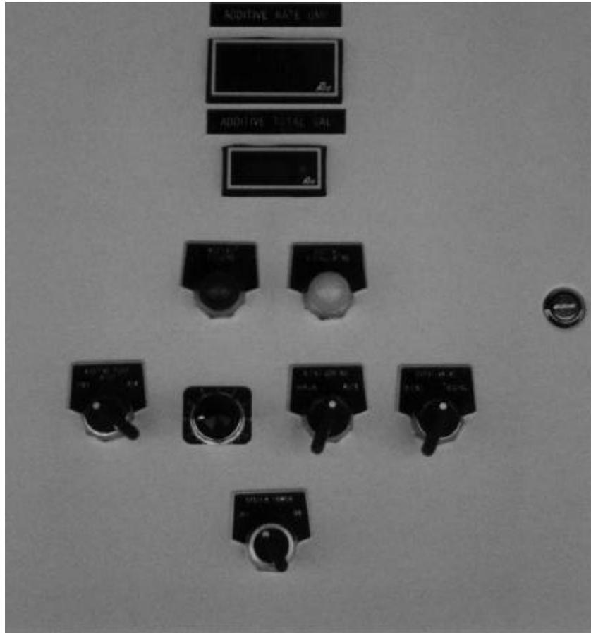
Figure 4.31 Batch plant liquid additive control panel.
