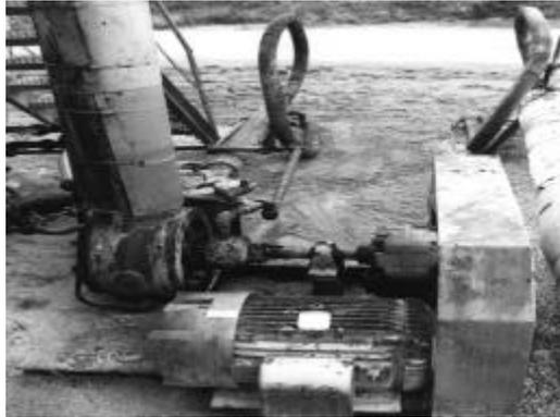
Figure 4.17 Asphalt tank off-loading pump.
