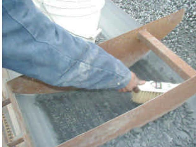
Figure 3 - Cleaning fines from belt.
