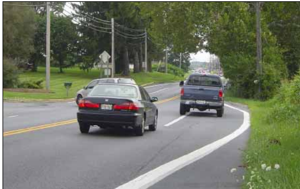
Figure 2.5 – Bypass lanes that eliminate the shoulder can impede bicycle travel Source: SHA's Application and Design Guidelines for Shoulder Bypass Lanes
