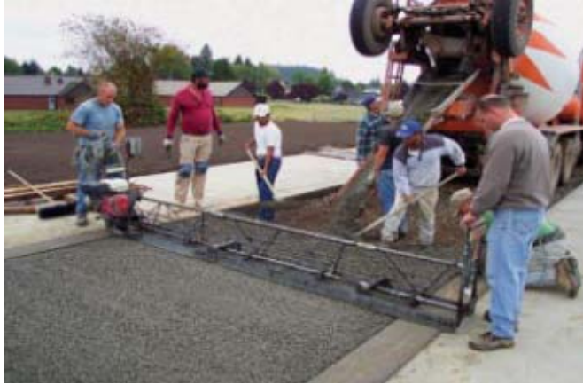
Figure 2.13: Mechanical Vibrating Screed
