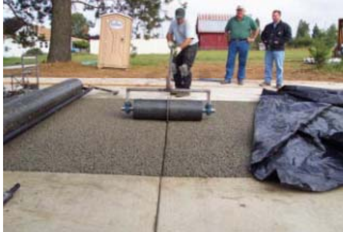
Figure 2.15: Use of a Rolling Joint Tool
